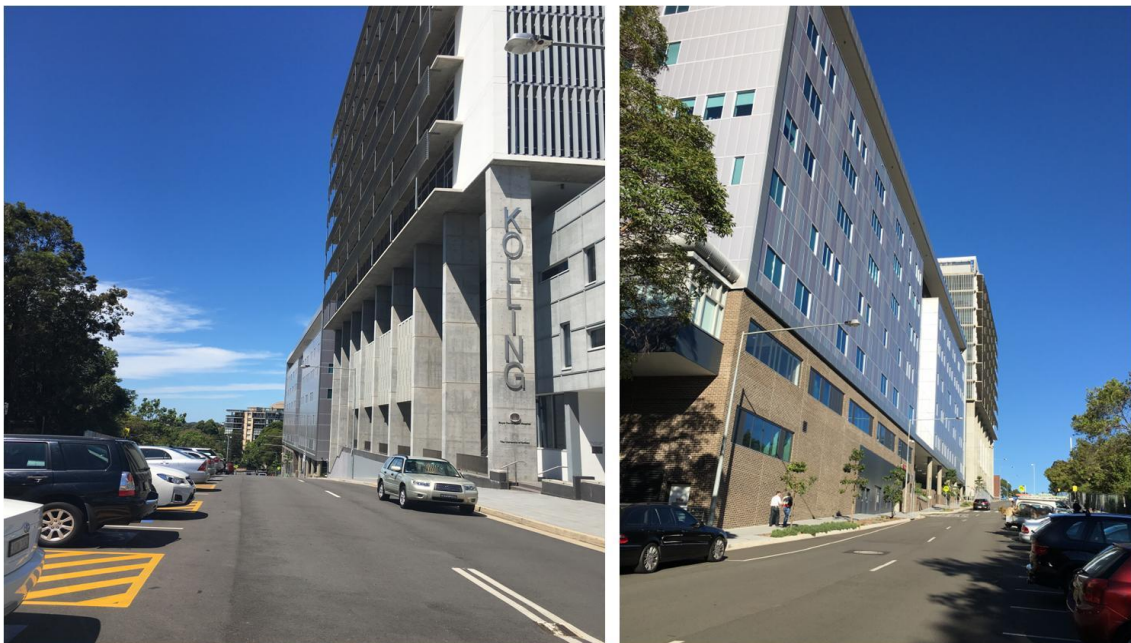
Figure 5: View looking east along Westbourne Street including the Kolling Institute to the south of the site (left) and view looking west along Westbourne Street including the Royal North Shore Hospital Clinical Services Building (right) (Source: KEYLAN Consulting)
