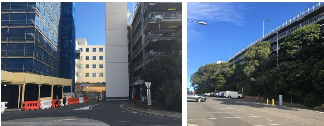
Figure 6: View west towards Royal North Shore Car Park and North Shore Private Hospital beyond (left) and view looking south along Reserve Road, with Royal North Shore Hospital car park to the west (right) (Source: KEYLAN Consulting)
