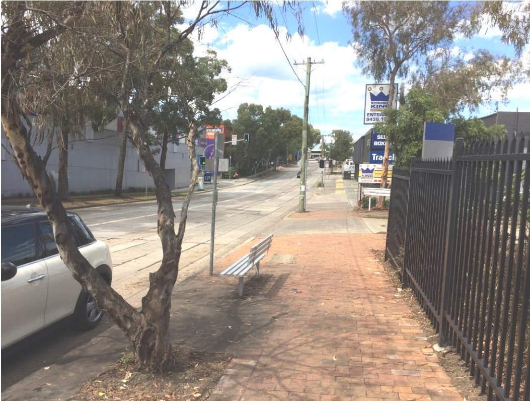
Plate 5: Looking east (downstream) from the Frederick Street Entrance/Exit towards the sag point in Frederick Street.
