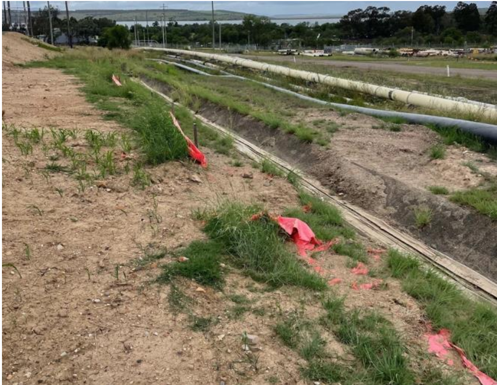
Plate 1 Sediment fencing requiring maintenance on the Stage 1 site while ground cover develops
