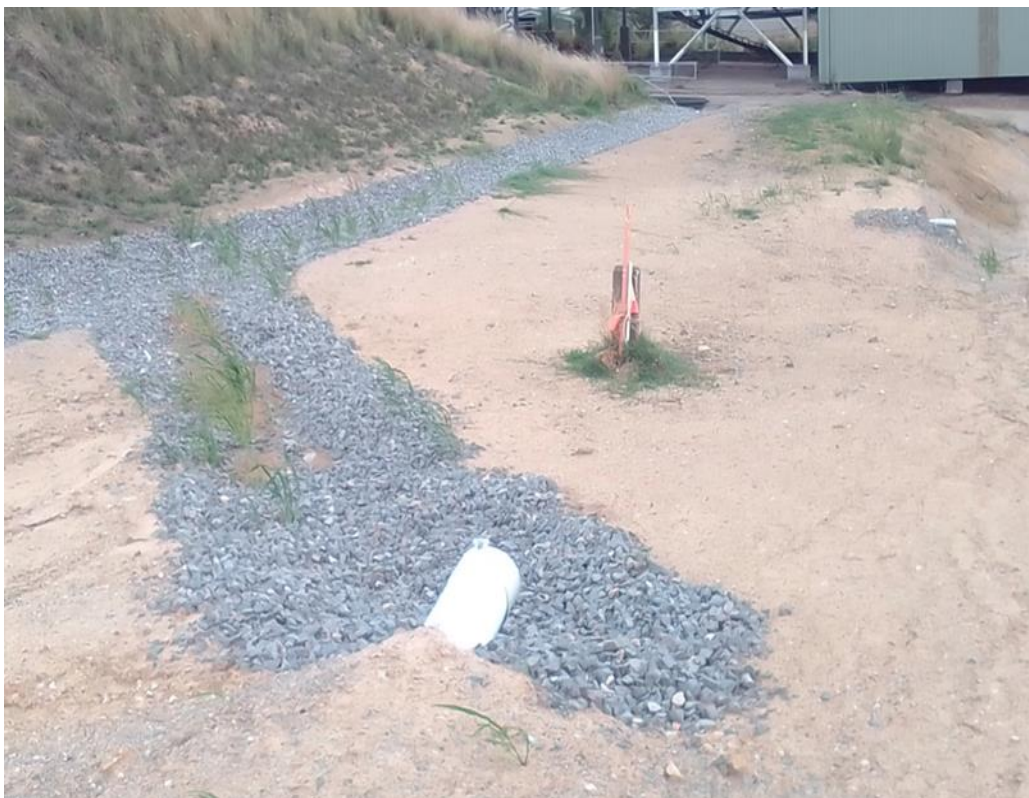
Plate 4 Erosion and sediment control measures available on the Stage 1 site and some exposed areas requiring reseeding
