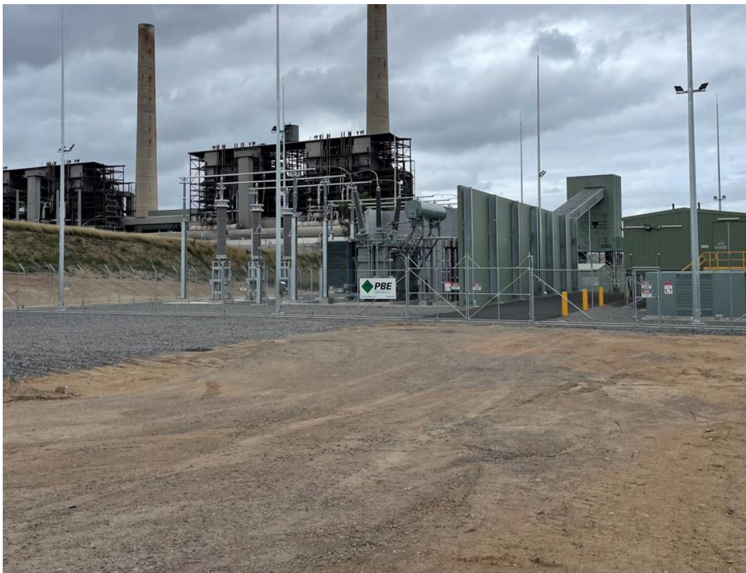
Plate 10 Stage 1 Project area, with low dust emissions. Permanent infrastructure is clad to minimise visual contrast.
