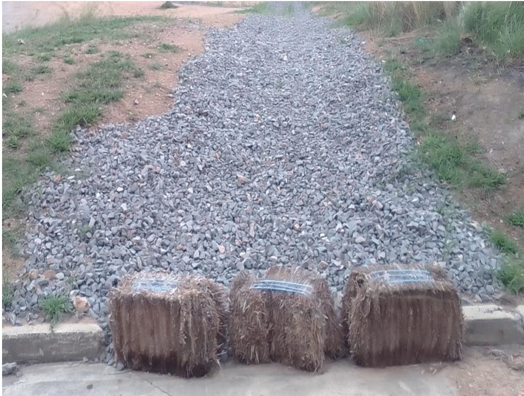
Plate 3 Erosion and sediment control measures available on the Stage 1 site
