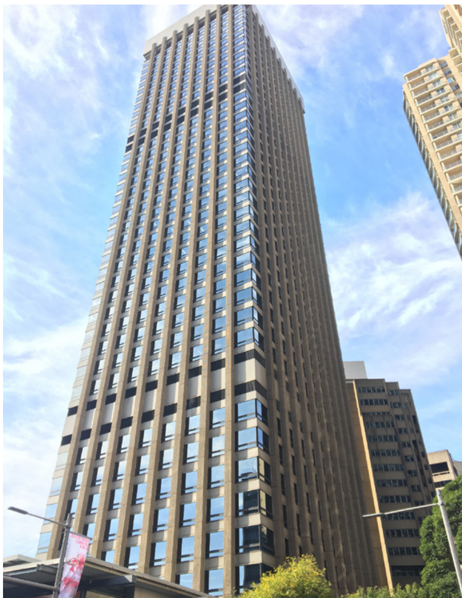
Figure 28 – Existing development at 201 Elizabeth Street
