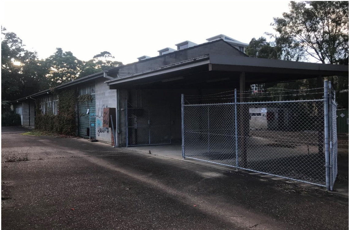
Photograph: 1 Vacant buildings
