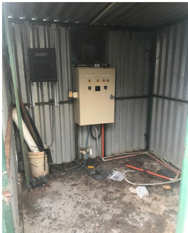
Photograph: 22 Shed (formerly for pump equipment?)
