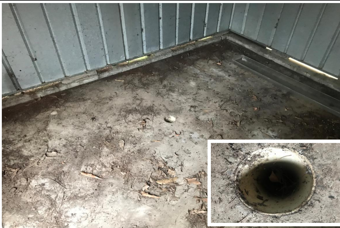
Photograph: 15 Eastern chemical store metal shed, concrete floor, with vertical conduit
