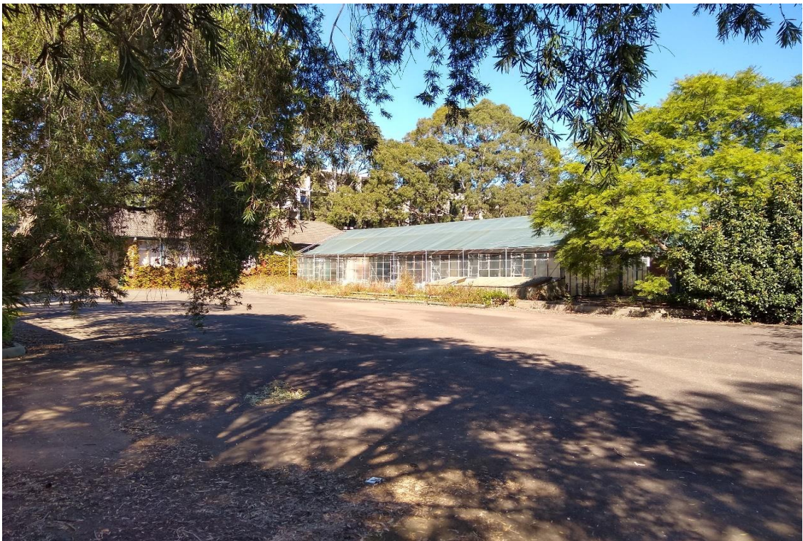
Photograph: 4 Paved road and greenhouse in northeast part of site
