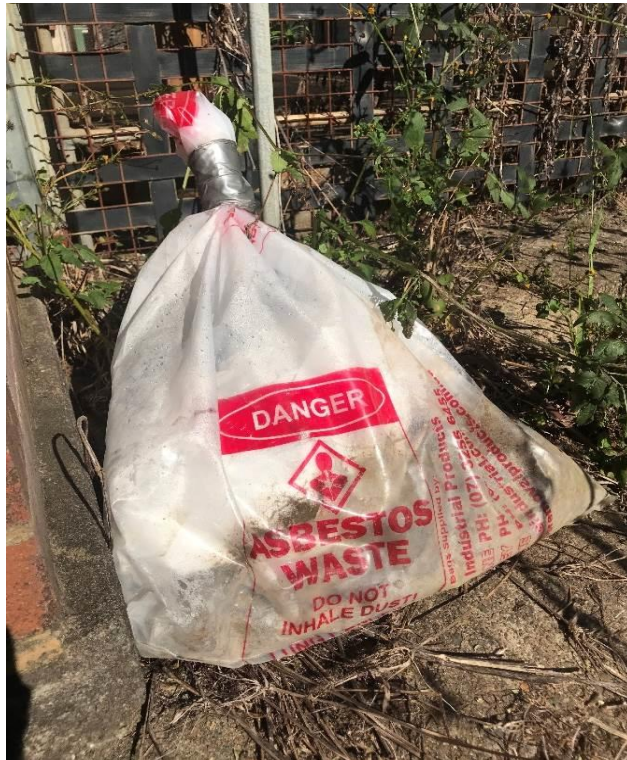
Photograph: 27 Bagged Asbestos near Oxidizing Agent Store
