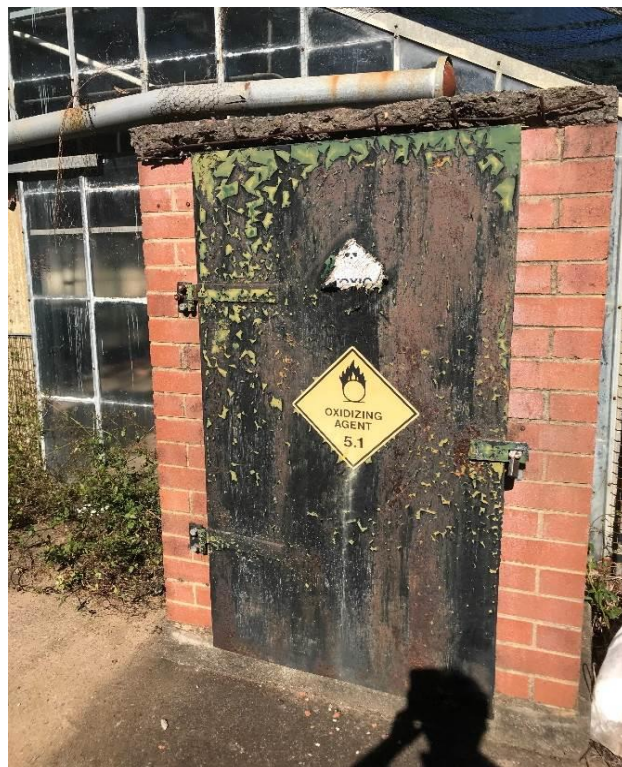
Photograph: 24 Oxidising Agent Store
