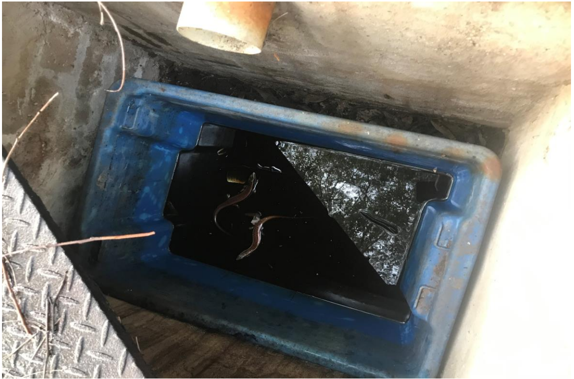
Photograph: 17 Oily substance in plastic container in pit from previous photograph, possibly from conduit
