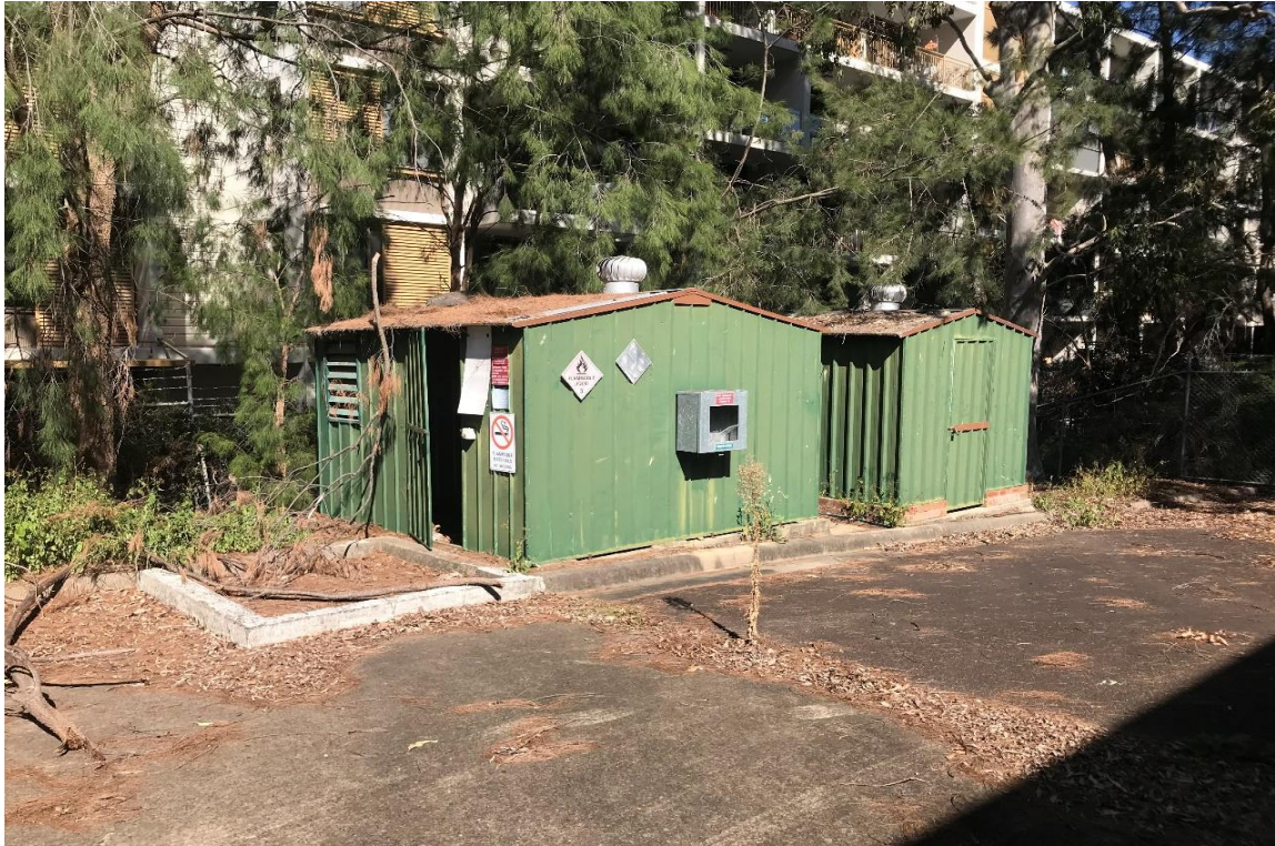
Photograph: 11 Metal sheds apparently used for chemical stores, with adjacent possible bunded area.
