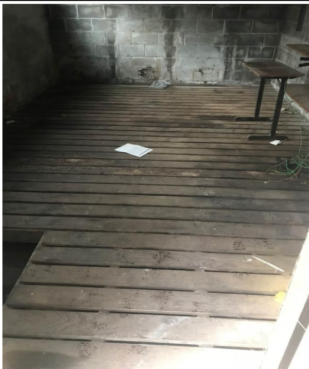
Photograph: 9 Besser Block Flammable Goods Store - wooden floor boards with some dark staining and corner of sub-floor access
