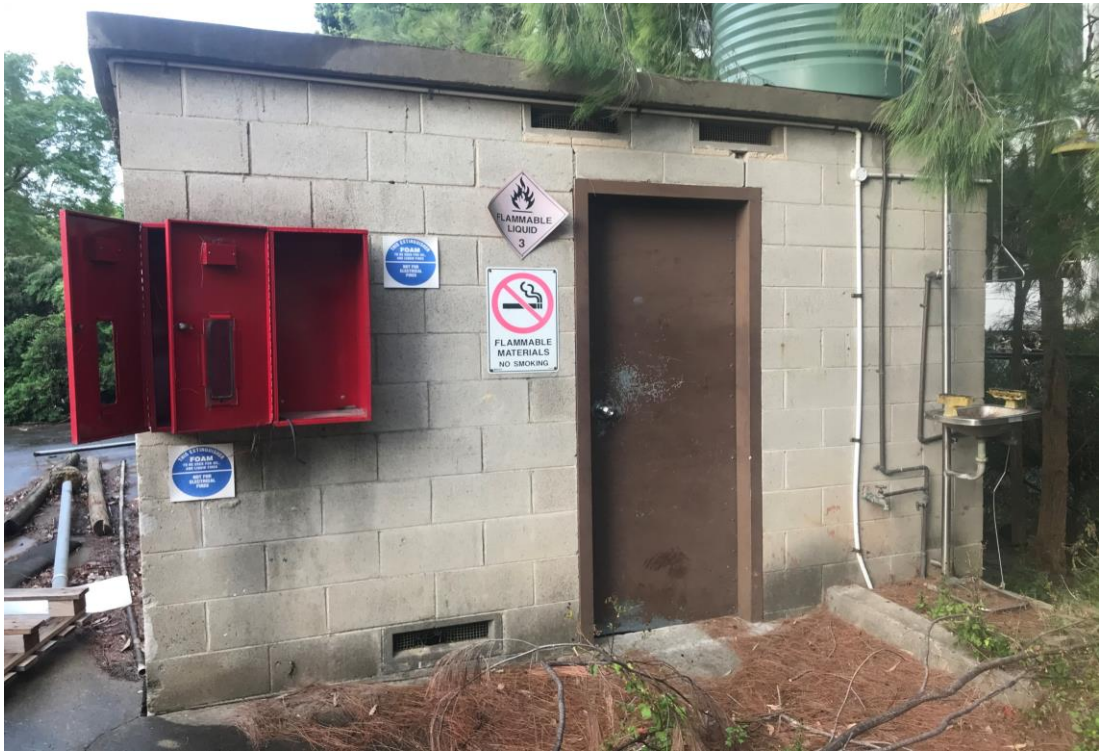
Photograph: 7 Besser Block Shed labelled with Flammable Goods (Flammable Goods Store)
