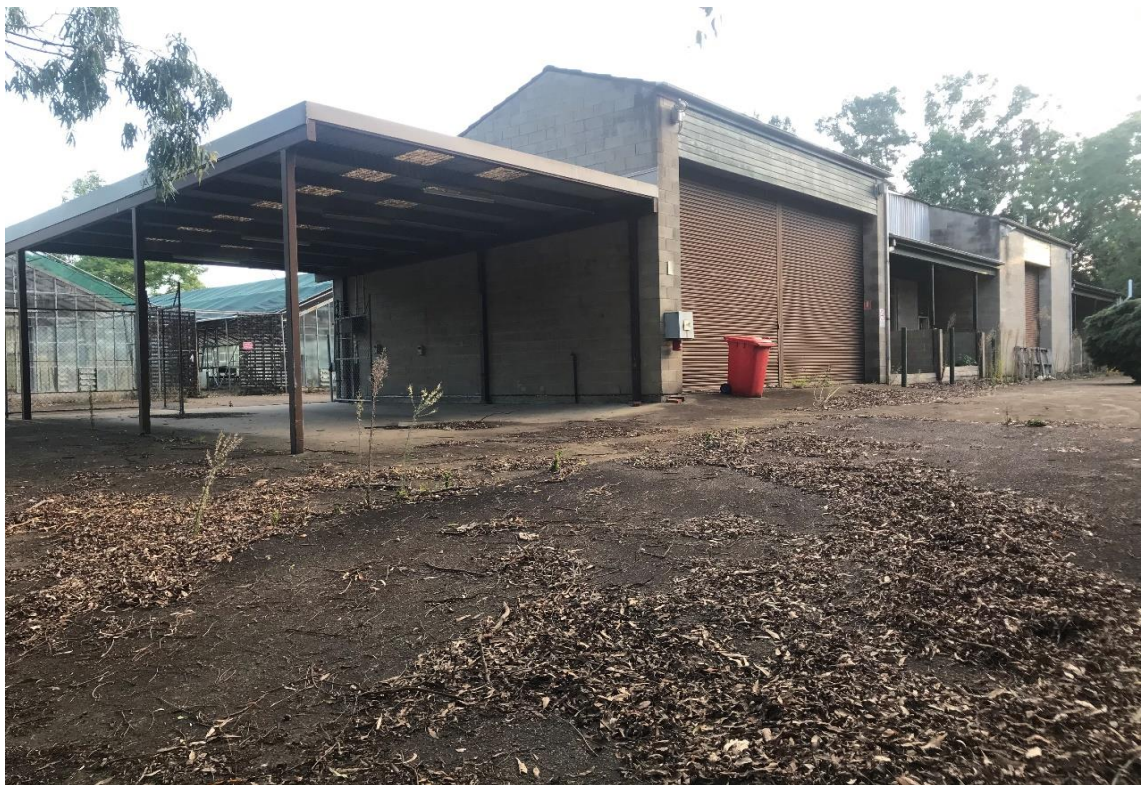
Photograph: 2 Vacant buildings
