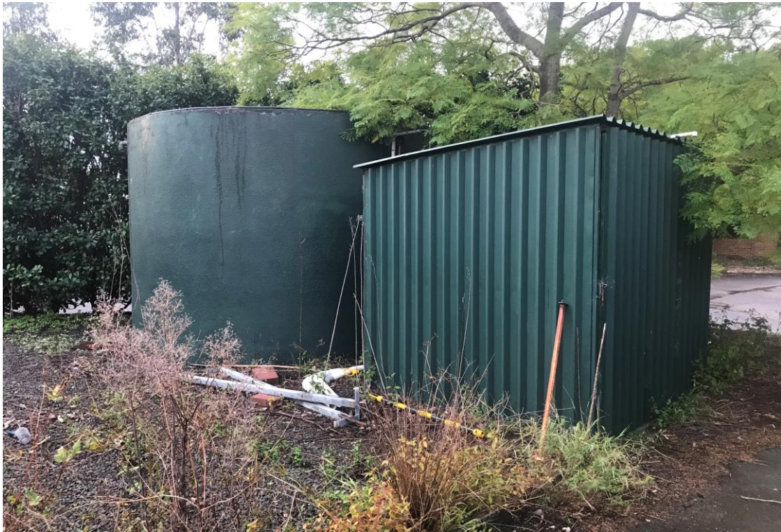
Photograph: 21 Water tank and shed (formerly for pump equipment?)
