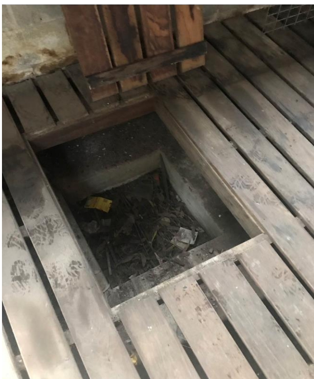
Photograph: 10 Besser Block Flammable Goods Store - hatch in wooden floor with underlying concrete slab (with cut out)
