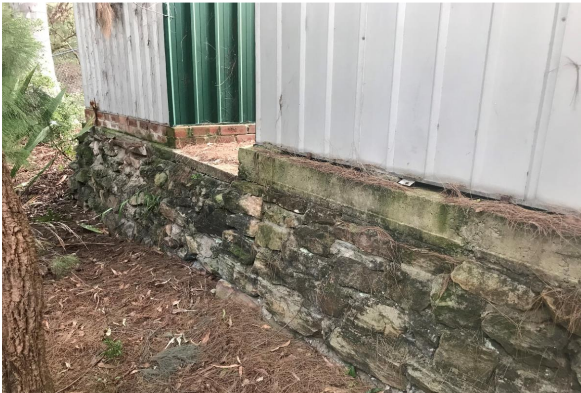
Photograph: 12 Southern side of the chemical store metal sheds, showing retaining wall
