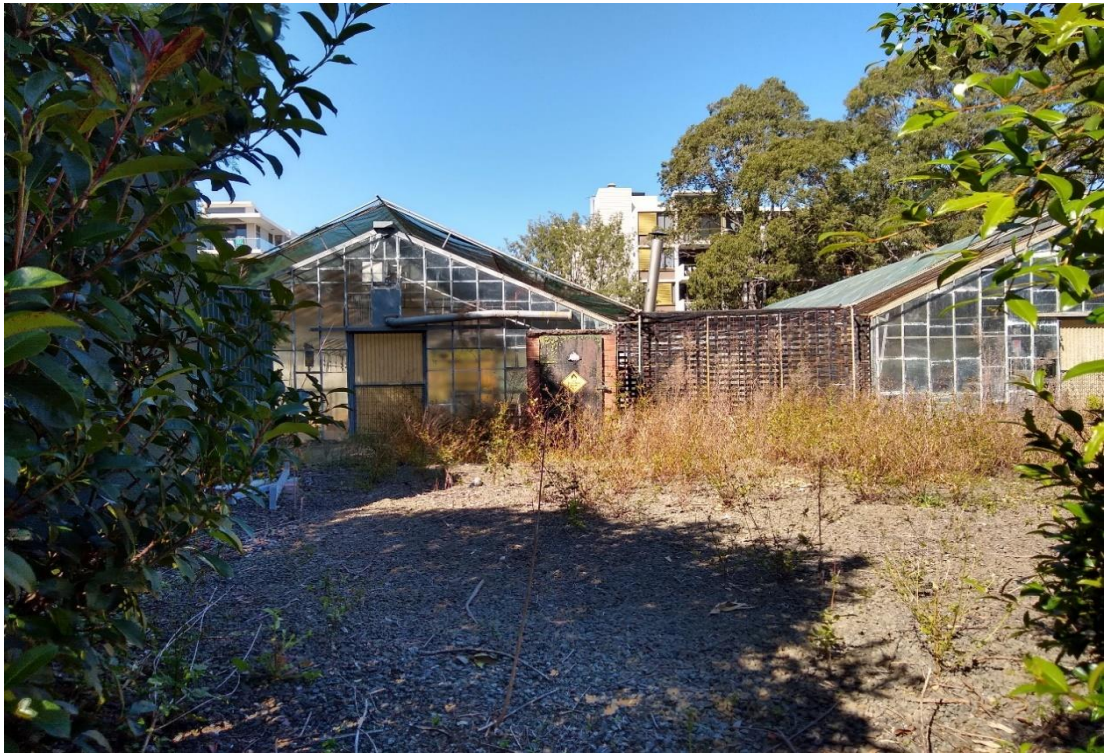
Photograph: 23 Greenhouses with Oxidising Agent Store
