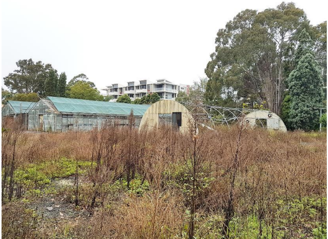
Figure 9 Existing glasshouses to be demolished. Epping Park development in the background
