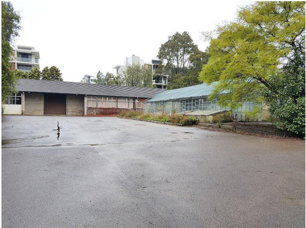
Figure 4 Looking south towards existing TAFE buildings to be demolished. Residential apartment buildings associated with Epping Park development in the background
