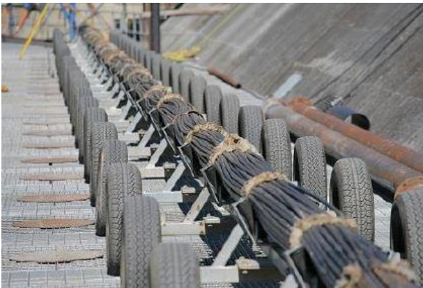
Figure 2-6 Example trolleys conveying tendons
