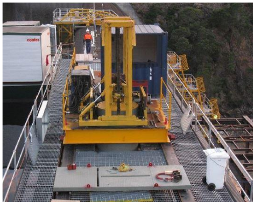
Figure 2-3 Example of coring rig on dam crest
