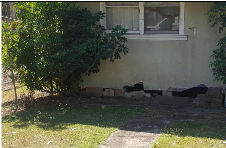
Photograph 15: Photograph showing the dilapidated building constructed of fibre cement sheeting, located in the south-west section of 135 Tenth Ave.
