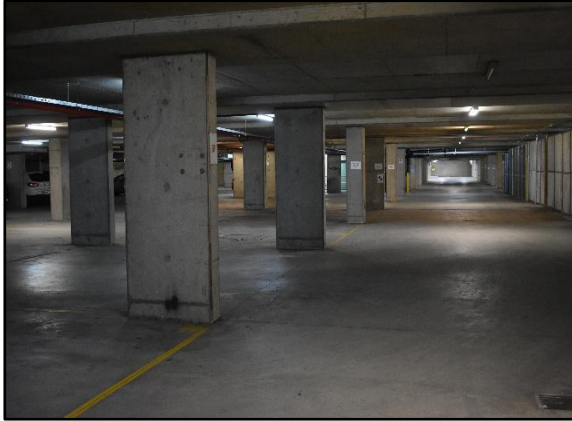
Figure 32: Basement-level carpark facing north
