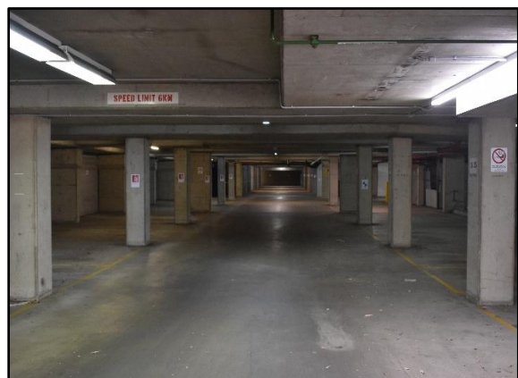
Figure 31: Basement-level carpark facing south
