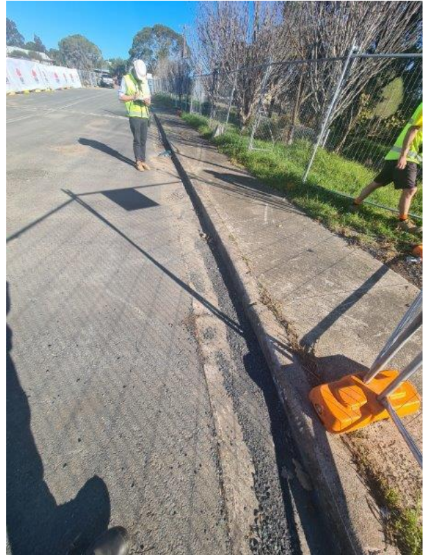
Figure 6: Accumulation of gravel and dirt in gutter
