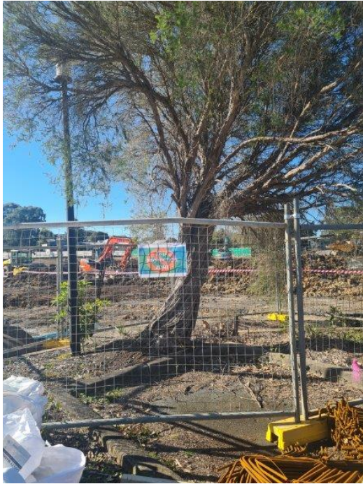
Figure 1: Tree protection measures
