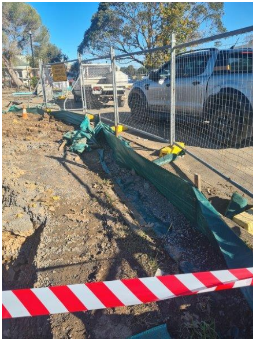
Figure 3: Sediment fencing installed and requiring maintenance
