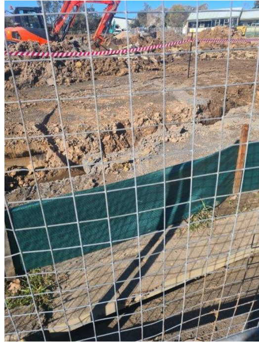
Figure 2: Sediment fencing installed
