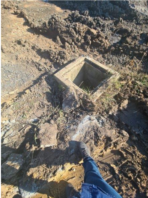
Figure 5: Stormwater pit containing sediment, erosion and sediment controls not installed
