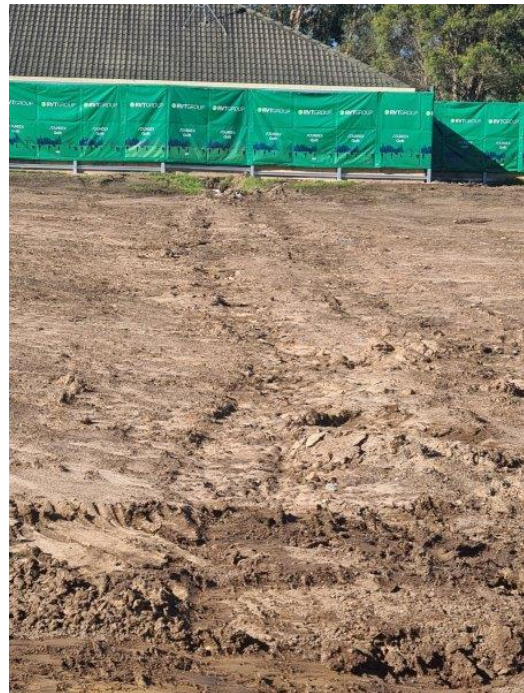
Figure 4: Hoarding for noise mitigation
