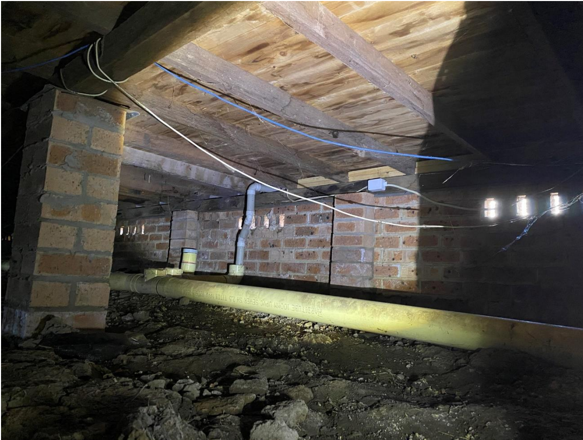
Figure 10: Underfloor area, Block M
