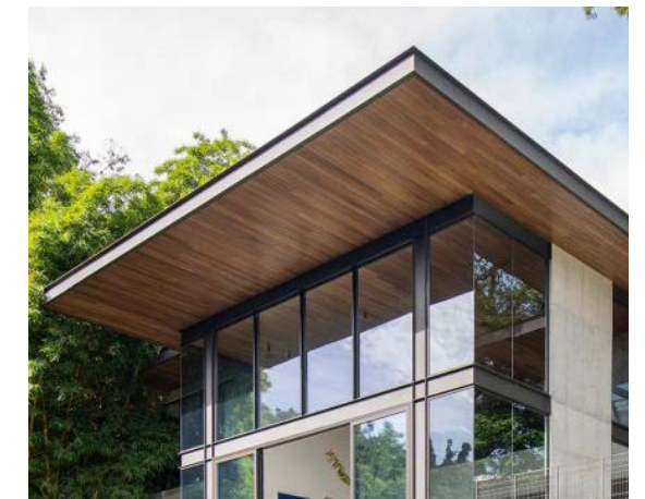
Oversailing roofs with timber effect soffit and exposed structure
