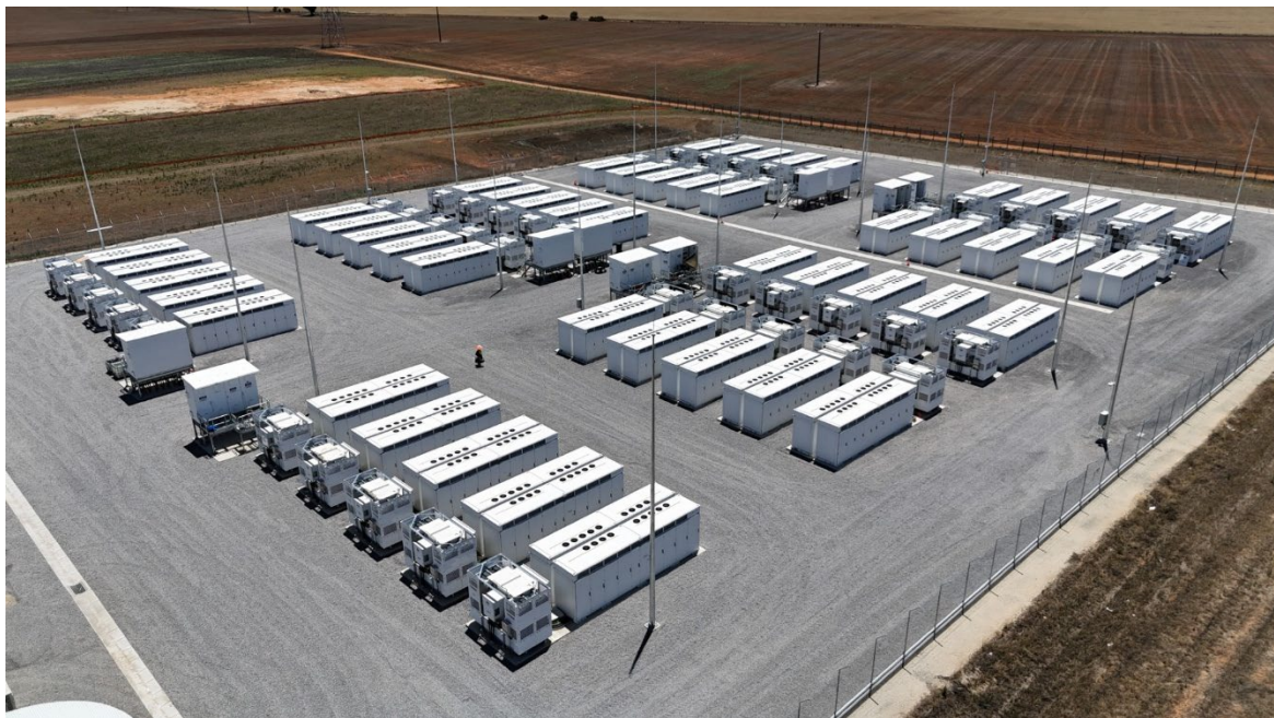
Figure 7: Indicative BESS Project layout (Edify Koorangie BESS)
