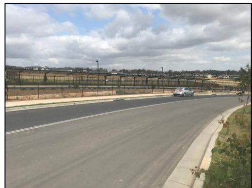
Figure 13: View of existing bus bay along Jardine Dr (Source: CPSD)
