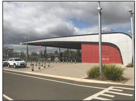
Figure 29: Edmondson Park Railway Station at the south-eastern side of SFCC (Source: CPSD)
