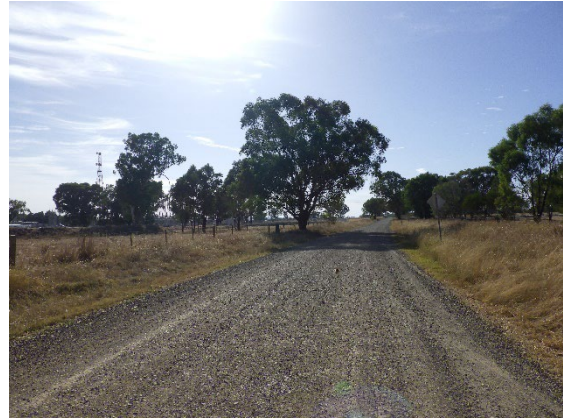
Figure 5 – Boiling Down Road (view east)
