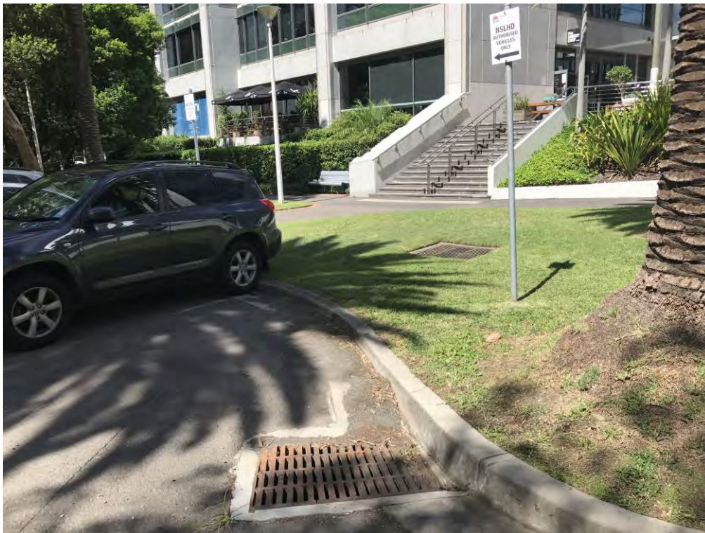
Plate 6: The existing grated inlet pit (Pit 4) located in the south eastern corner of Site 4A that is directly connected to the 900 mm trunk drainage line
