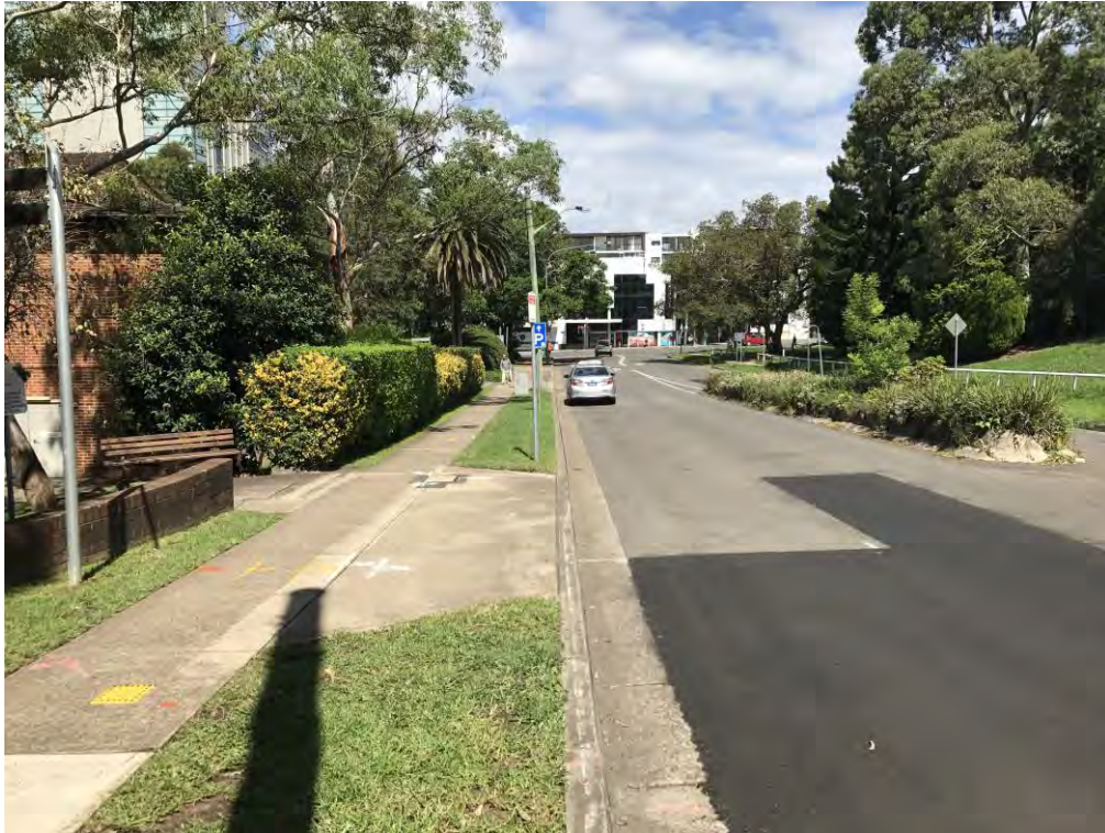
Plate 3: Looking south (downslope) from the northern boundary of Sites 4A and 4B along the eastern side of Reserve Road.
