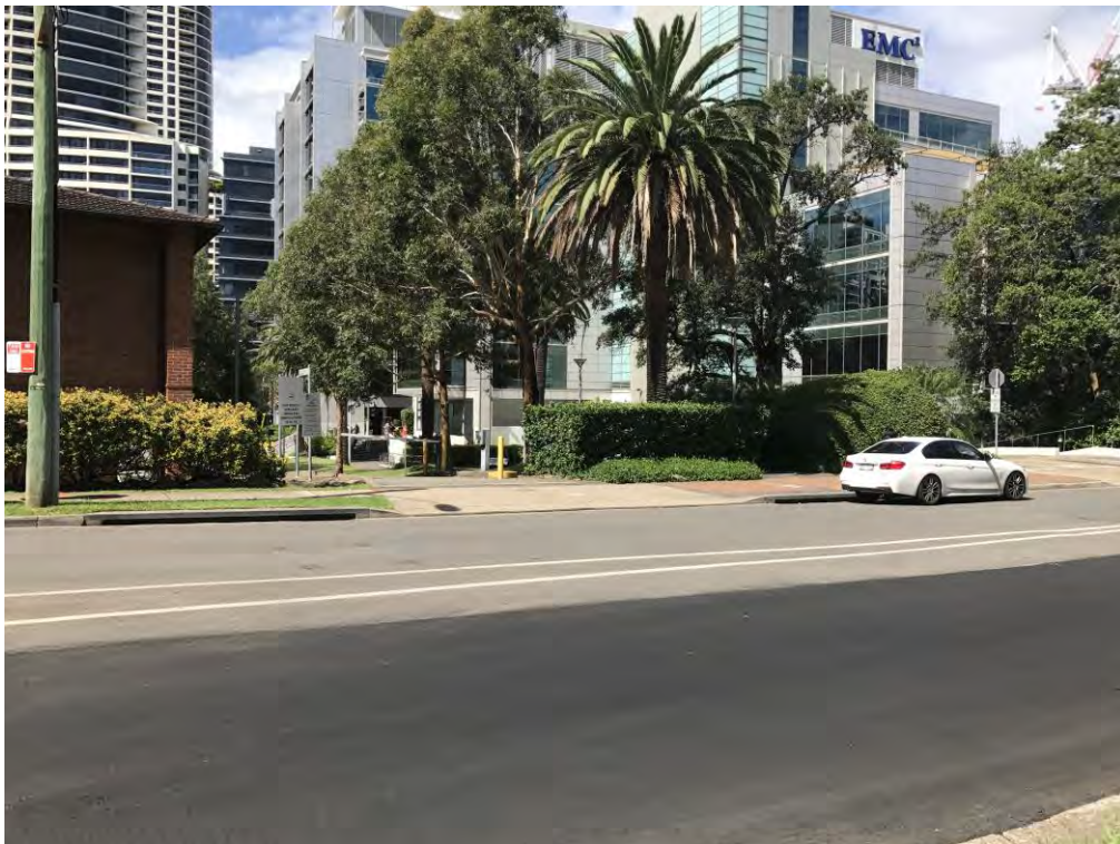
Plate 4: Looking east (downslope) towards Sites 4A and 4B from Reserve Road at the Existing Reserve Road Driveway Entrance.
