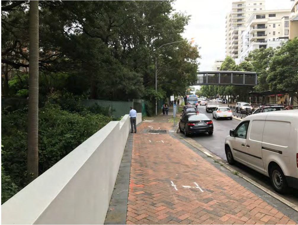
Plate 9: Looking north (downslope) along the existing concrete wall along the Herbert Street frontage of the trapped low point in Lot 11 DP1013030.
