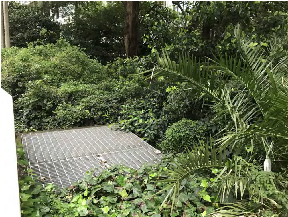
Plate 8: The large grated inlet structure (Pit 7) which is located in the trapped low point in Lot 11 DP 1013030.
