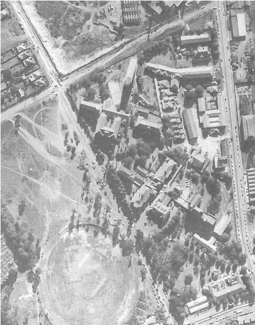
Figure 9.15 1961 aerial photograph of the RNSH. Sturt House (Building 6) had been completed by this date, and the Laundry (Building 19) had been constructed adjoining the 1925 Mortuary. Just south of the Mortuary, along Herbert Street, the new boiler house (Building 21) was one of the new facilities to be erected during this period of growth. Note that the land on the western side of Reserve Road is as yet undeveloped.
