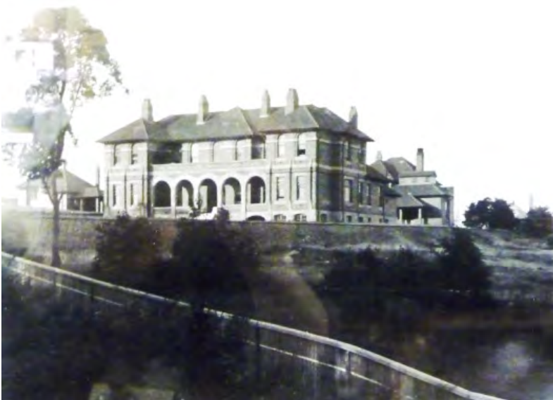
Figure 4.2 View of the Administration Block (Building 31), set within its embankment. The Operation Block can be seen on the left, the Kitchen Block can be seen on the right (Building 33)
