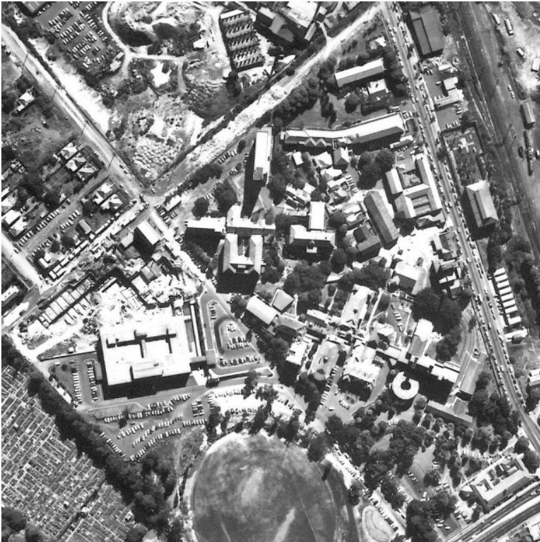
Figure 10.1 1972 aerial photograph of the site. By this date, the Western Precinct has been developed, as has the CJ Cummins Building (34) and the Child Care Centre (Building 38) on the eastern side of the site.
