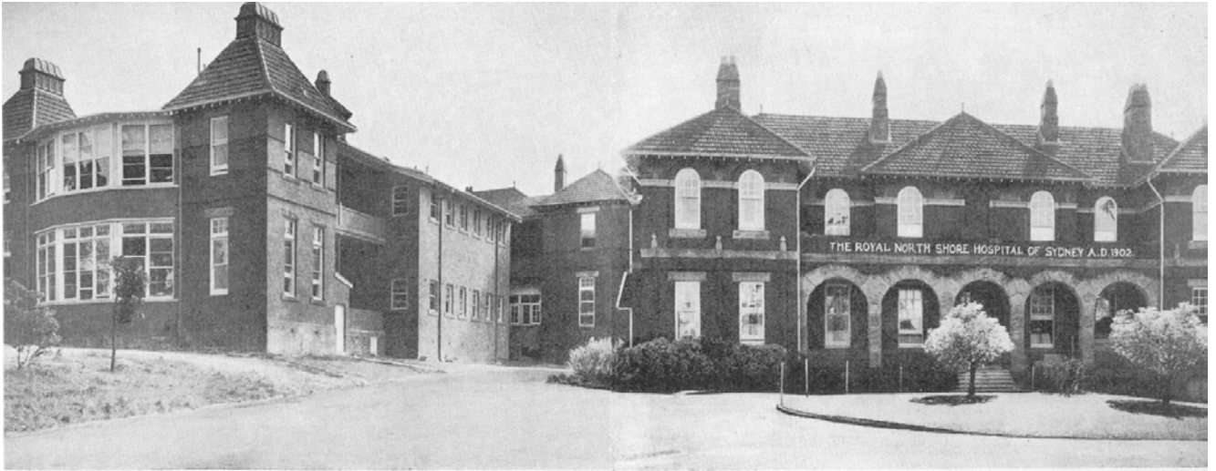
Figure 9.9 Building 30 (left) after remodelling, and Building 31 (right) 1950. Note glazed projecting solarium at the end of the Building 30 and the changes to the verandah Source: RNSH Museum
