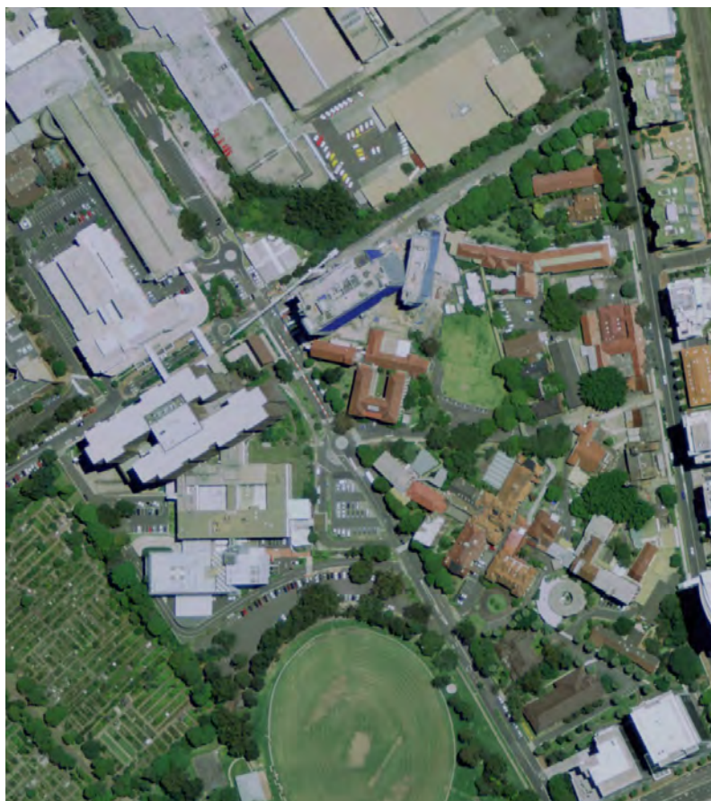
Figure 11.7 The initial stages of redevelopment: the north-western corner of the block bounded by Westbourne Street and Reserve Road, with the new Kolling Building in course of construction
