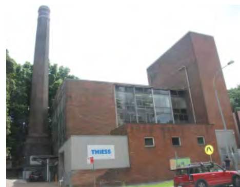
Figure 3.4 Building 21 and the redundant chimney on the eastern side of the Original Hospital Precinct, viewed from Herbert Street
