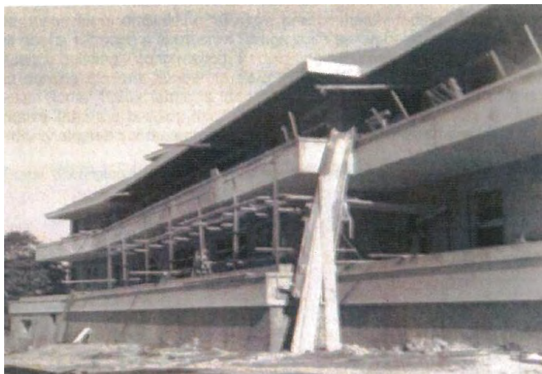
Figure 9.16 Building 10 under construction, 1947 Source: RNSH Archives
