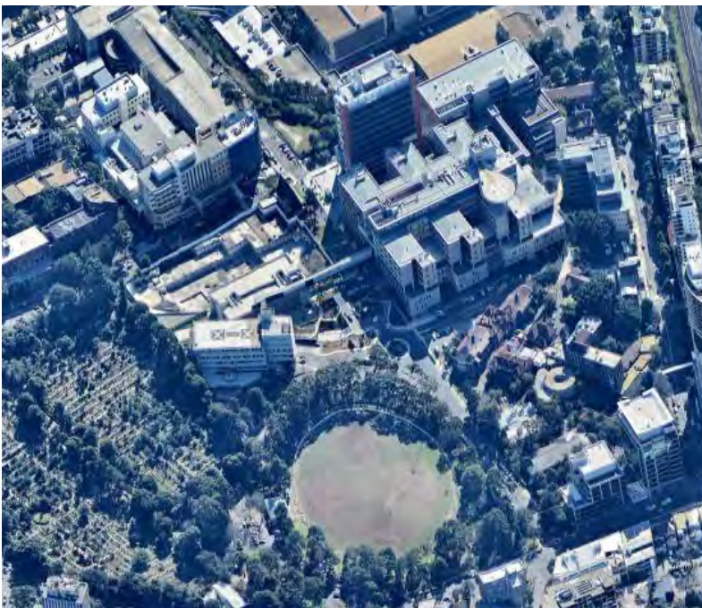
Figure 11.10 2016 north view showing the demolition of Main Blocks 1 and 2 on the western side of Reserve Road, following the transfer of patients to the new hospital block
