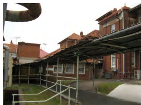
Figure 3.3 View of the eastern side of the Original Hospital Precinct showing the former Waiting Room, (Building 32) between the Kitchen Block (Building 33) and the Pavilion Wings (Buildings 29 and 30) and the covered walkways
