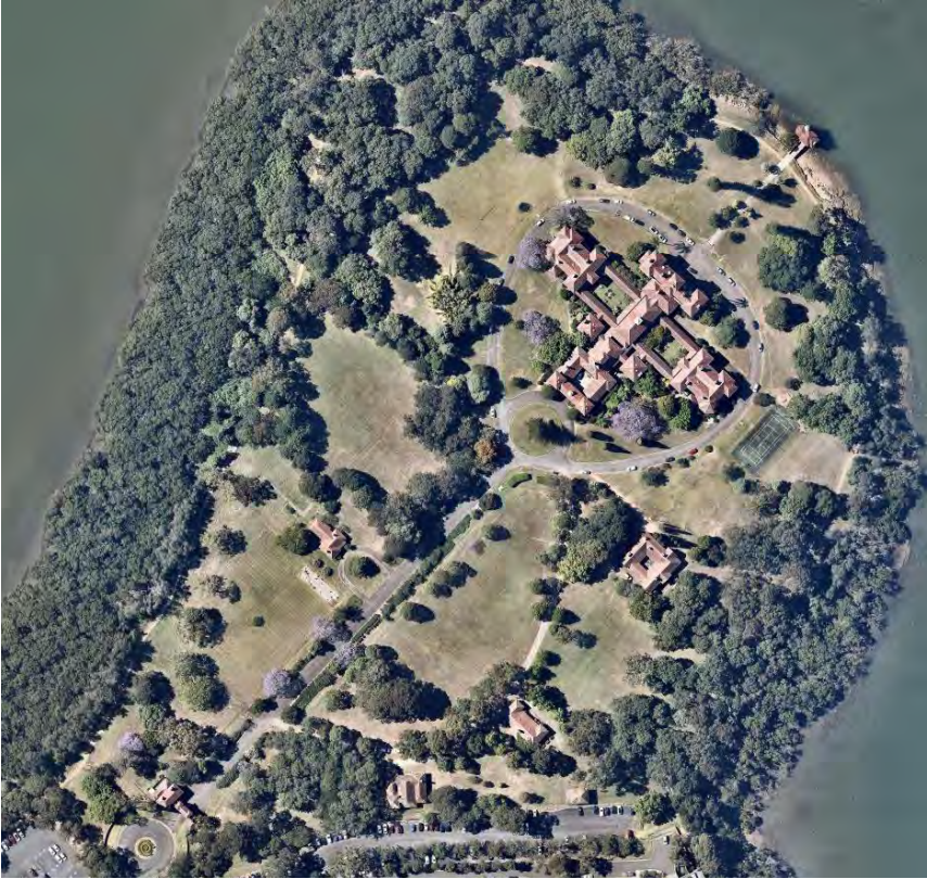
Figure 5.3 Aerial photograph showing the Thomas Walker Convalescent Hospital Precinct
