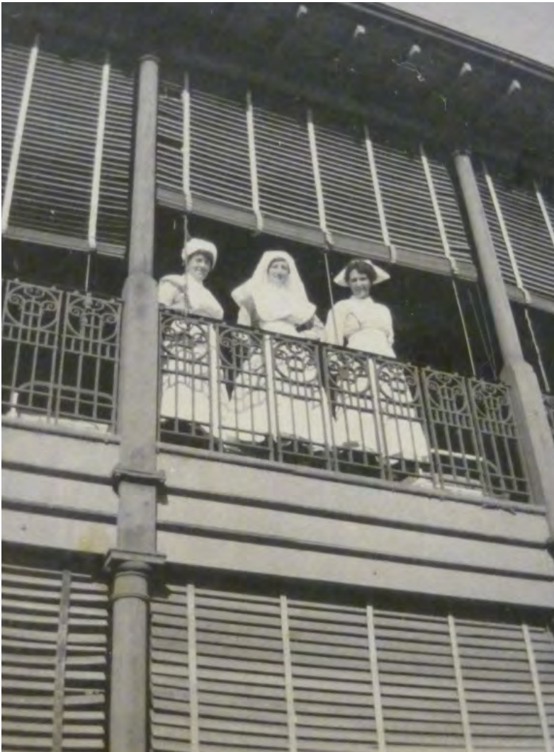
Figure 6.5 Photograph showing the verandah and eaves details of Building 30, circa early 1920s
