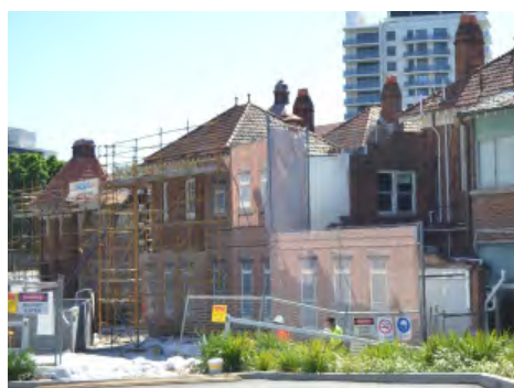
Figure 3.13 The junctions of buildings attached to the north of Buildings 29 and 30 were retained when they were removed and are currently screened with printed fabric to improve the aesthetic
