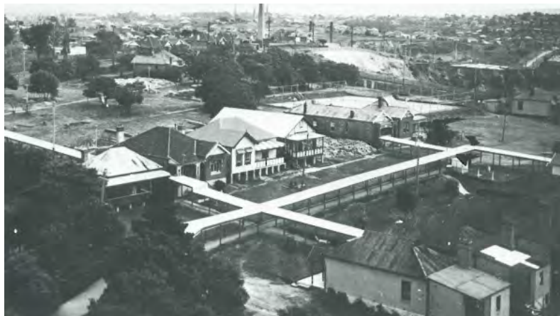
Figure 6.9 Resumed cottages adapted for use as maternity wards and nursing staff accommodation
