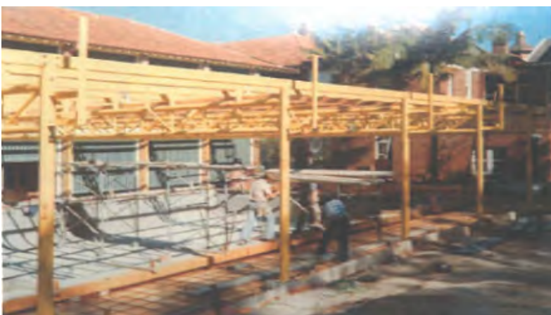
Figure 10.3 Hydrotherapy (Building 28) under construction, 1977 Source: photograph by Peter Priestly (RNSH Collection)
