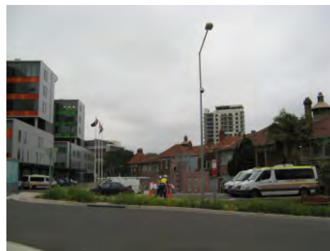
Figure 3.12 The original pavilion wings (Buildings 29 and 30) have lost their context and setting through recent hospital redevelopment
