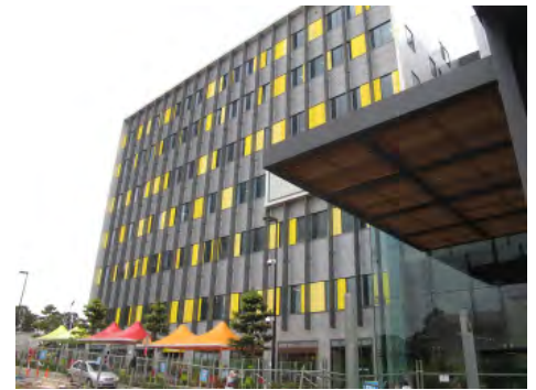
Figure 3.6 The Acute Services Building (Building 1) in the Northern Precinct
