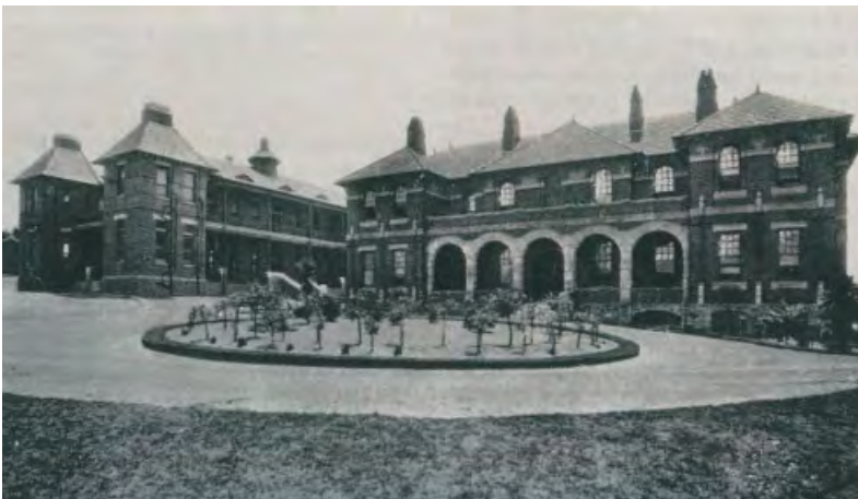
Figure 4.12 View showing the newly completed pavilion wing (Building 30) adjacent to the Administration Block (Building 31), c.1914
