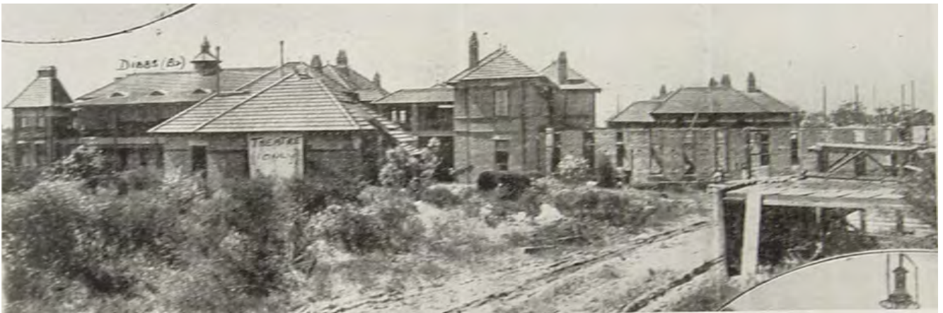
Figure 4.10 Construction of the second pavilion (later A Block/Building 30) c.1912. Note the completed annex of the 1912-1914 pavilion (centre) compared with the main body of the pavilion wing (right). Building 31 is visible beyond the construction of Building 30, the rear extension has been completed.
