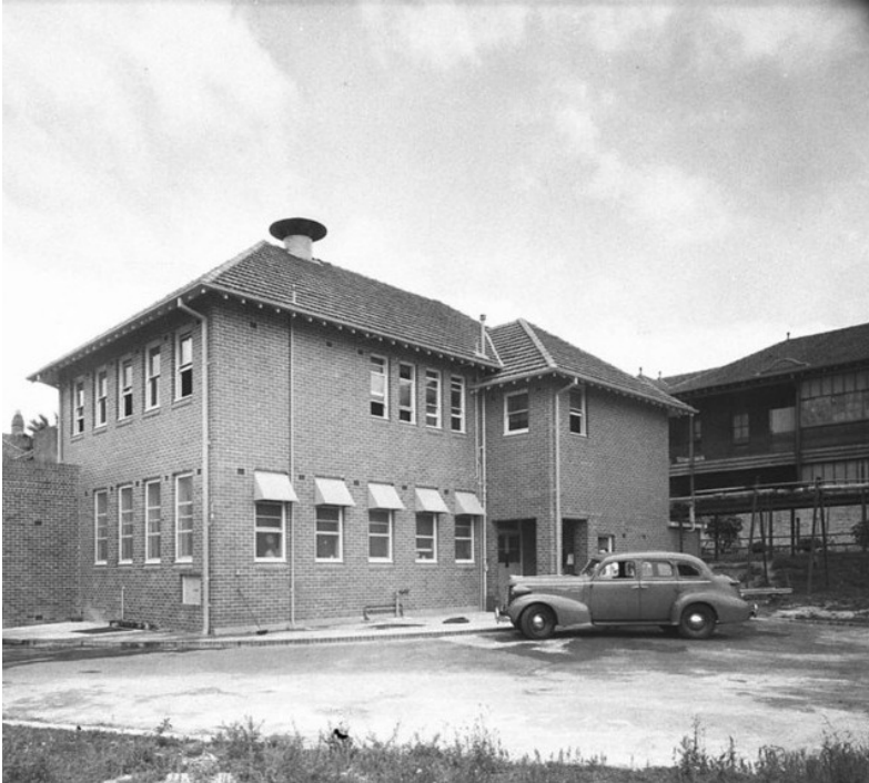
Figure 9.7 1950s photograph of the Kitchen (Building 33) recorded by Sam Hood, showing the rear extension.
