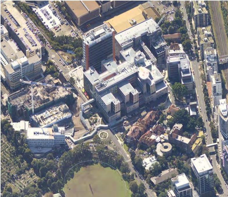
Figure 11.9 2013 view showing the deconstruction of the buildings on the eastern side of Reserve Road.
