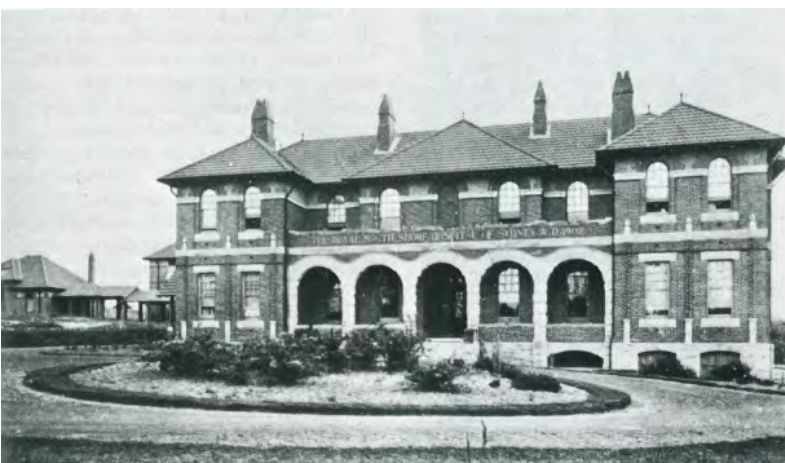
Figure 4.4 1905 photograph showing the main Administration Block and the original Operating Block at far left, which was demolished during World War II
