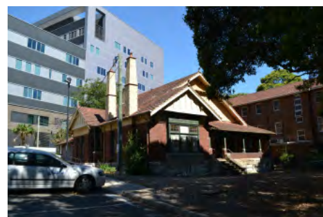
Figure 3.16 Building 9, Lanceley Cottage, at the Herbert Street frontage of the site, adjacent to the Clinical Services Building
