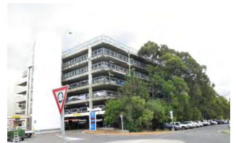
Figure 3.7 Car Park P1 in the North Western Precinct
