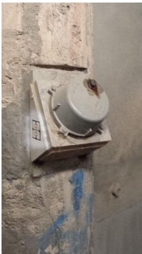
Example of access able anchor head
