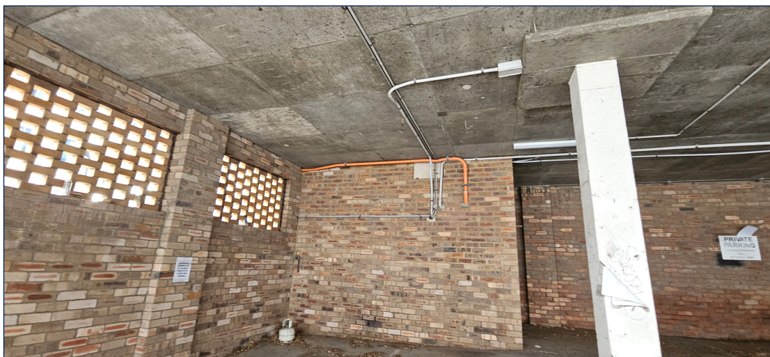
Figure 13. Under building carpark.
