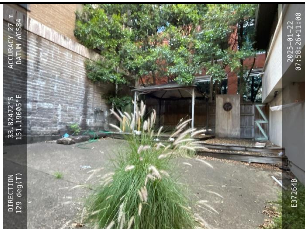
Photograph 8: Rear courtyard of 59 Christie Street.
