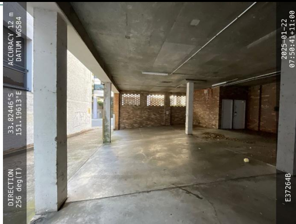
Photograph 4: The undercroft parking area along the lane between Nicholson Street and Christie Street.
