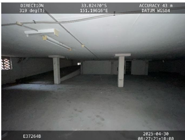
Photograph 6: Lower basement level of 46-48 Nicholson Street (along the south-eastern boundary of the site)
