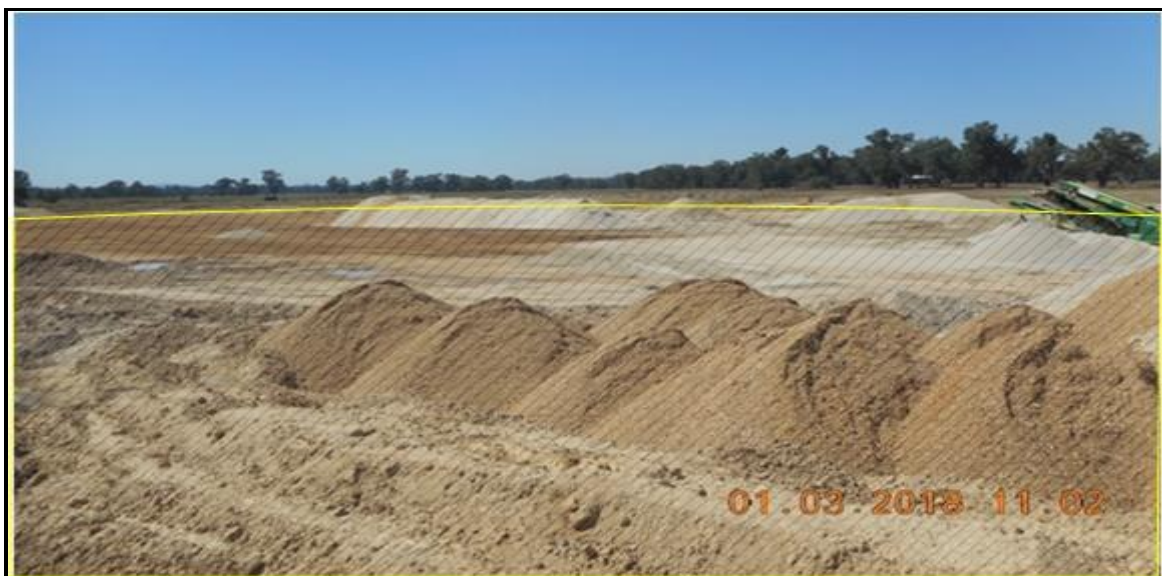
Figure 5 Quarry Site Stage 3 - View south
