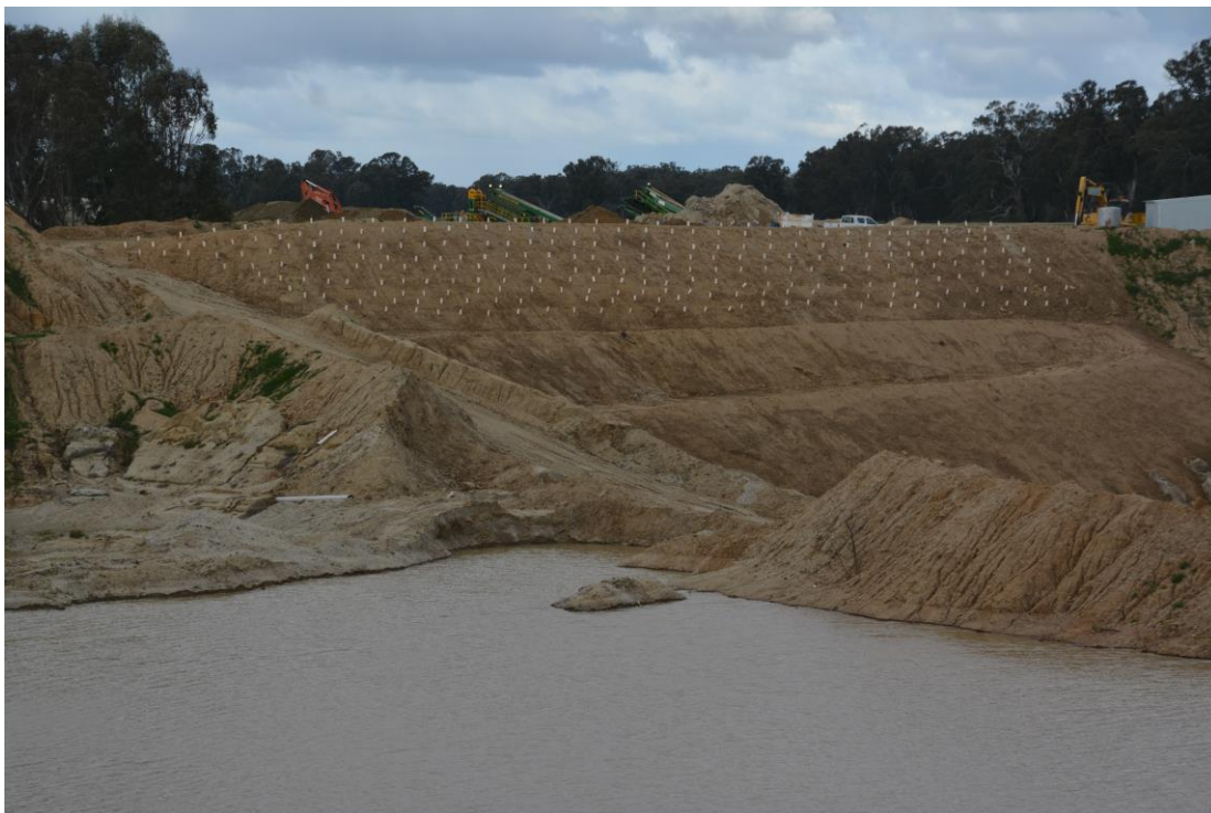
Plate 2.3 View of Existing Rehabilitation Profile and Revegetation (reference: E1019A_032)
