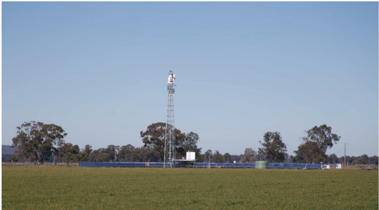
Figure 3.2 Tower and thermal receiver at Jemalong demonstration site viewed from north (photo: Vast Solar)
