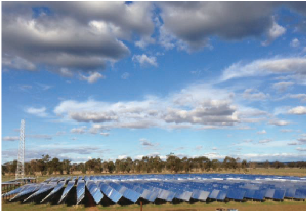
Figure 3.3 Heliostat fields at Jemalong pilot plant (photo: Vast Solar)
