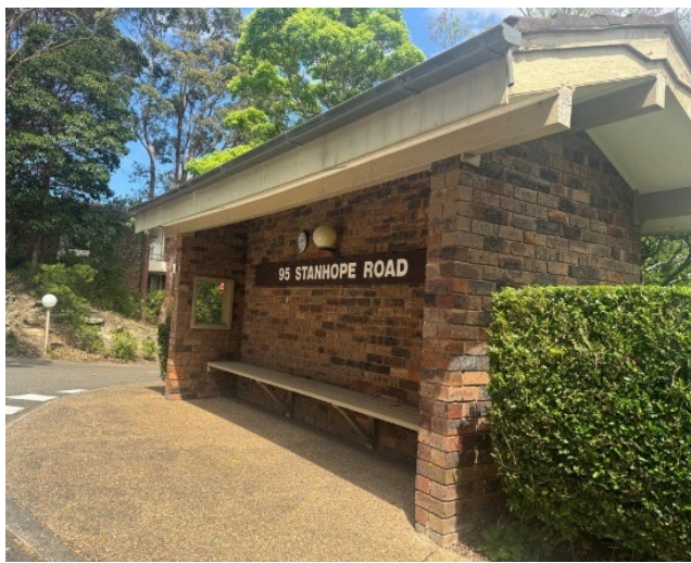
View of one of the existing bus stops on the site.
