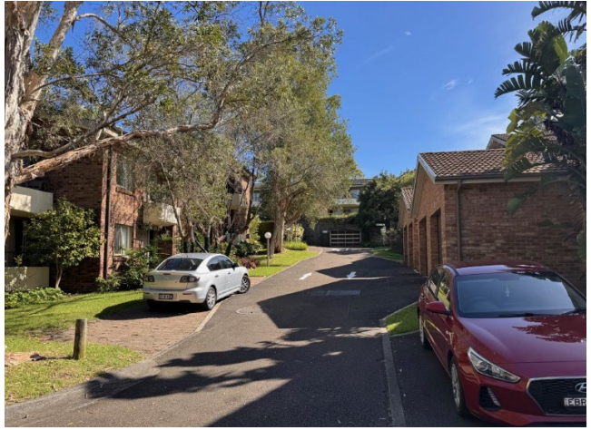
View within the site from Third Avenue looking north at the ILUs
