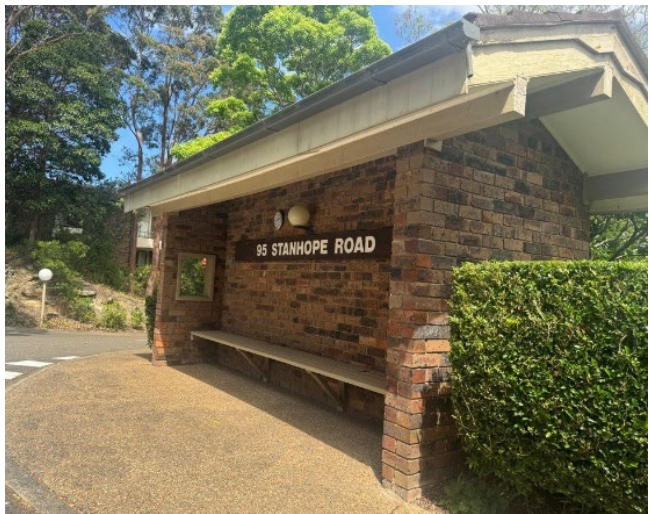
View of one of the existing bus stops on the site.
