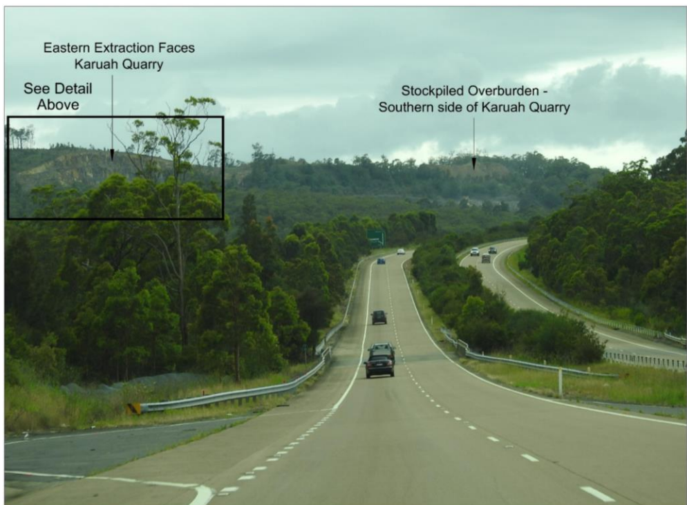
Plate 6.2 View to the east from the northbound lanes of the Pacific Highway towards Karuah Quarry (Ref: E958F_010)
