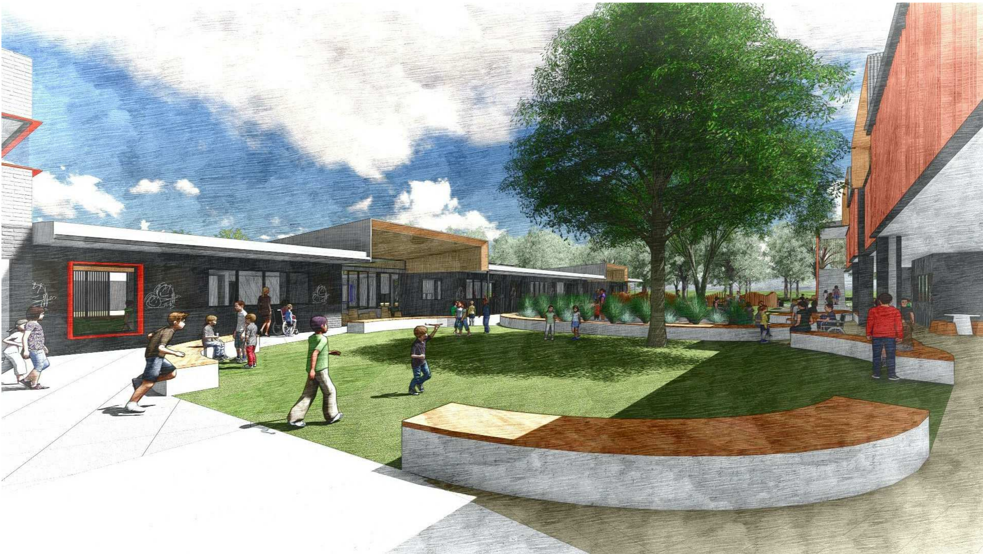
BLOCK C SOUTH FACADE FROM ENTRANCE
