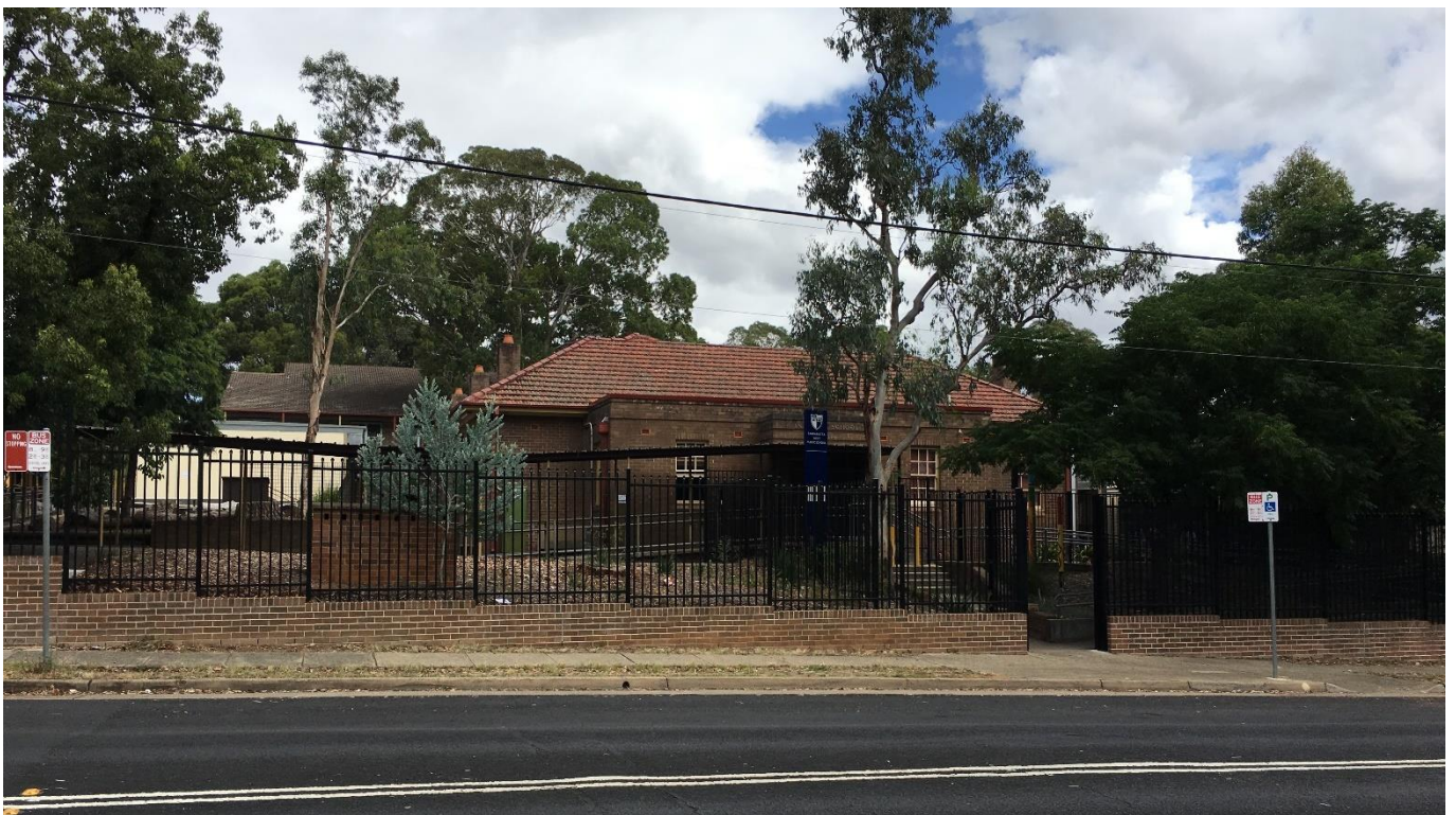
Photograph 2: Main school entrance from Railway Street
