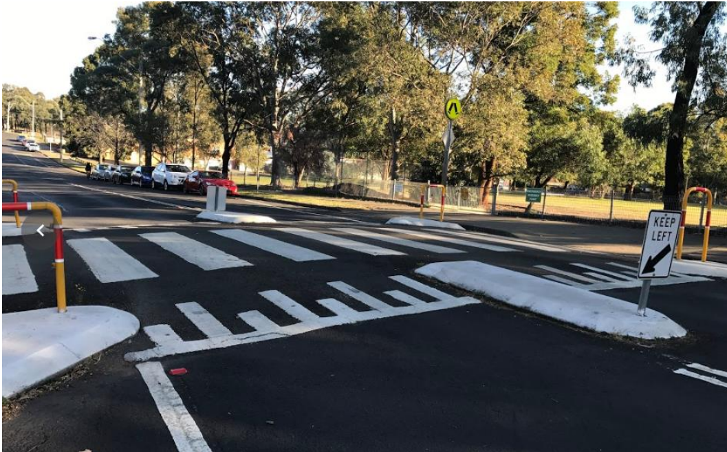
Figure 35: Raised zebra crossing connecting both buildings across Railway Street
