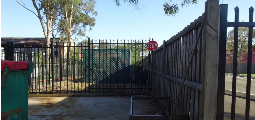
Figure 42: Existing loading area along Young Street
