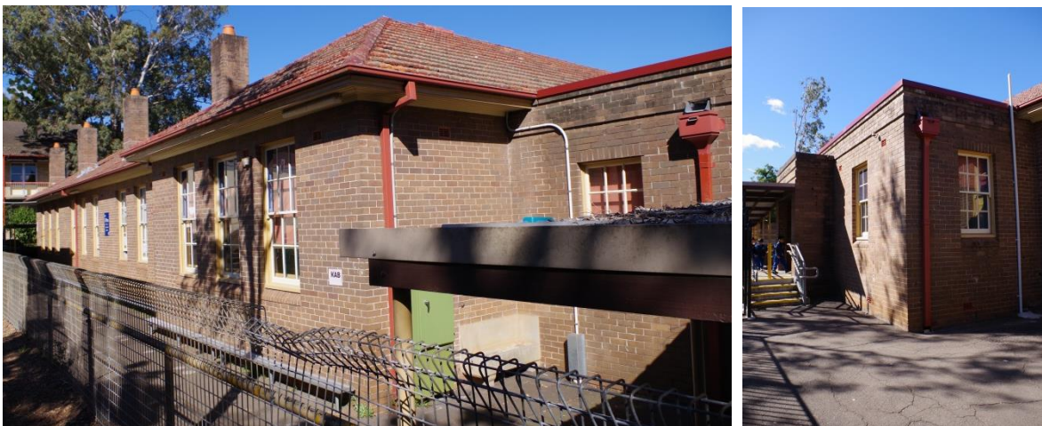
Figures 16 & 17: East façade (left) and the north-western corner (right) of building E. (Source: Conrad Gargett)
