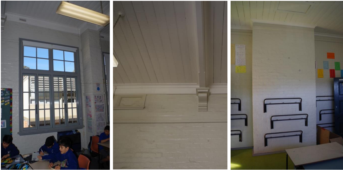
Figures 11, 12 & 13: Internal views of building F showing window towards south (left), timber board ceiling and decorative timber beam (middle) and fireplace (right). (Source: Conrad Gargett)
