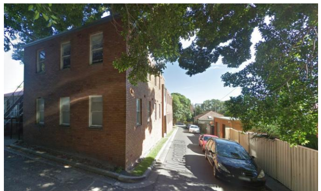
Figure 9 Maroubra Baptist Church office buildings, south of Maroubra Lane
