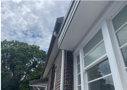
NS18: 133 Garden Street front exterior Eaves
