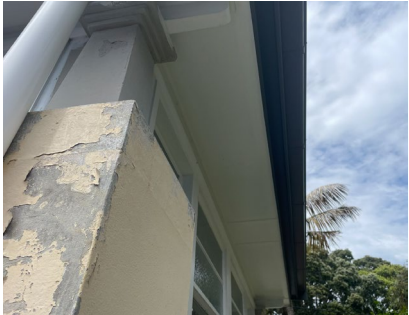
NS19: 133 Garden Street front veranda extension Eaves/ceiling
