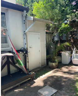
NS10: 255 Maroubra Road Extension exterior Exterior walls
