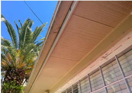
NS14: 257 Maroubra Road Exterior Veranda ceiling
