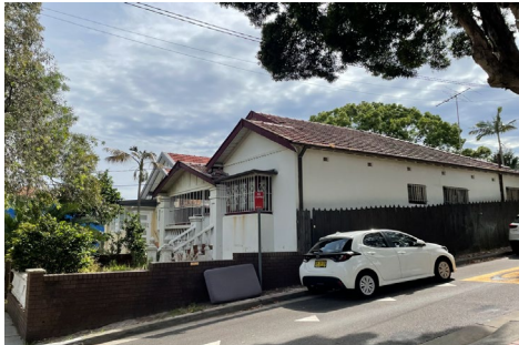
LS1: 135 Garden Street exterior Exterior walls
