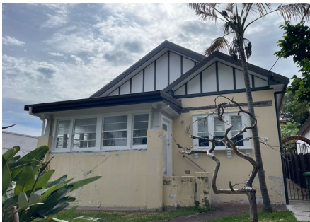
LS2: 133 Garden Street exterior Exterior walls
