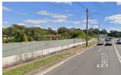
Beecroft Road existing condition
