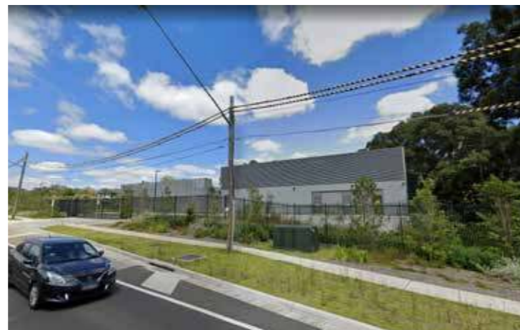
4 Sydney Trains Infrastructure
