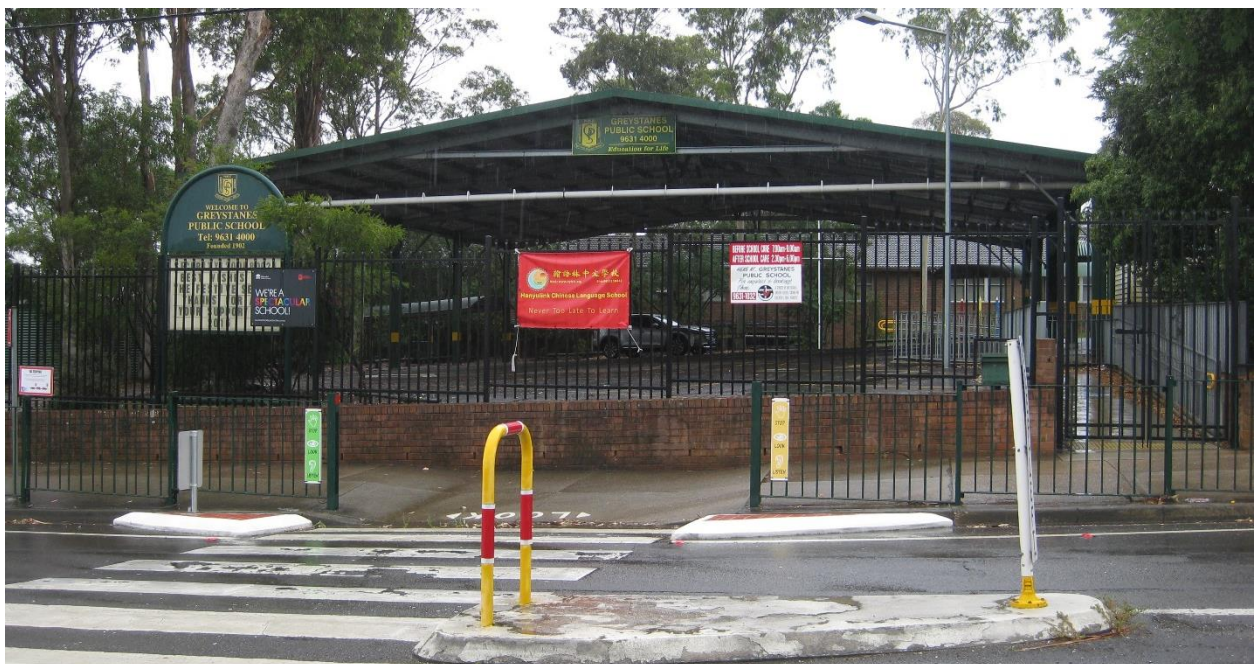
Figure 27 Existing entry is not visible or identifiable from the main entry
