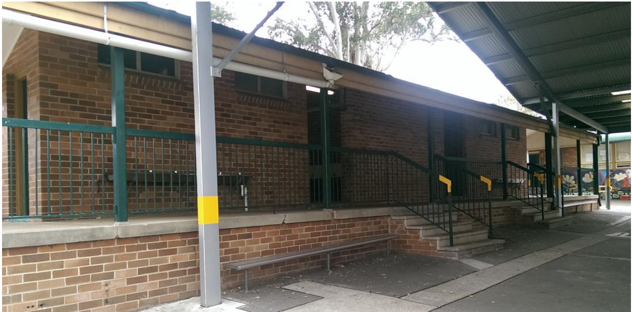
Figure 12 Block I – Existing amenities block
