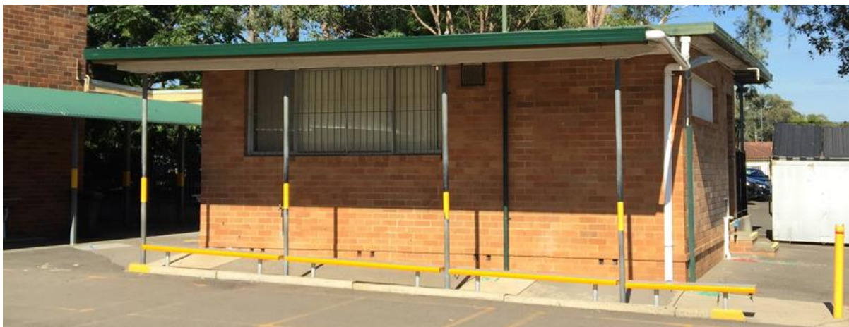
Figure 11 Block H – Existing garden store
