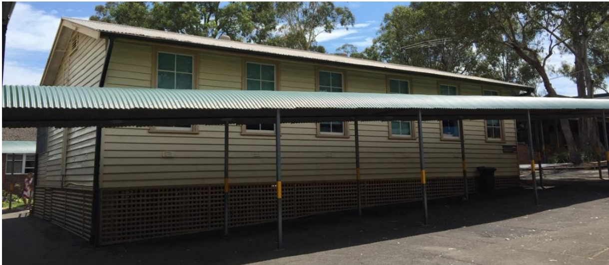
Figure 10 Block G – Former demountable
