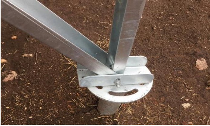
FIGURE 1 INDICATIVE SOLAR PANEL FOOTINGS
