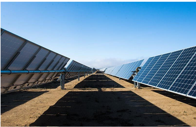
FIGURE 2 EXAMPLE OF TRACKING SOLAR PV PANELS
