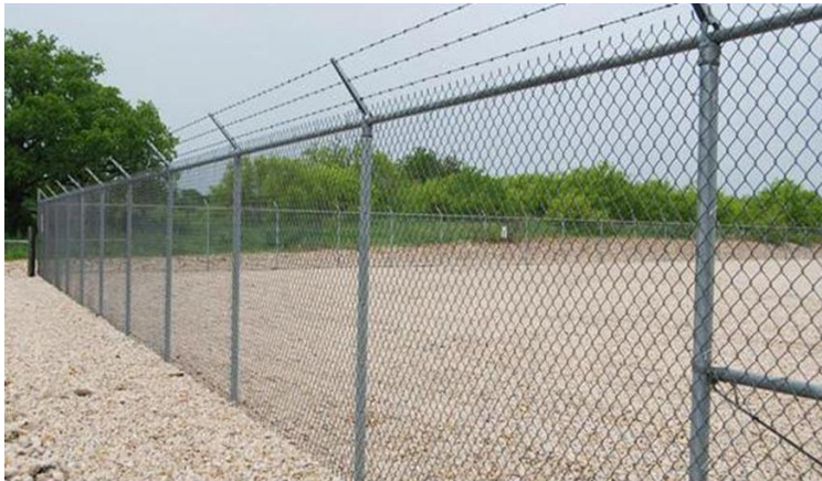
FIGURE 10 EXAMPLE PERIMETER FENCING
