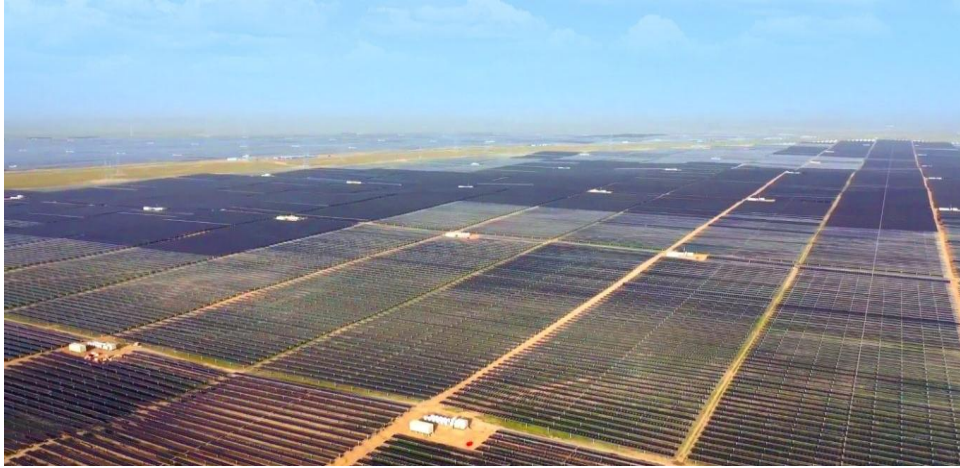
FIGURE 7 ILLUSTRATION OF BATTERY UNITS DISTRIBUTED THROUGHOUT A SOLAR FARM (SOURCE: HTTPS://EN.SUNGROWPOWER.COM/ )
