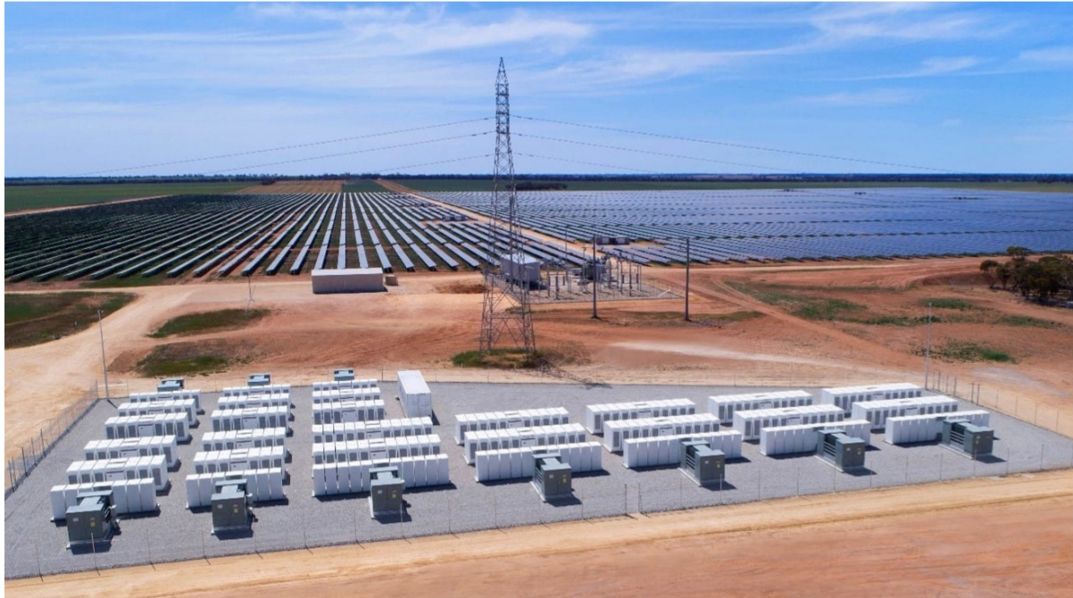
FIGURE 4 ILLUSTRATION OF A TYPE OF BESS COUPLED WITH A SOLAR FARM (SOURCE: WWW.ENERGYAUSTRALIA.COM.AU/ABOUT-US/ENERGY-GENERATION/GANNAWARRA-BATTERY-STORAGE )
