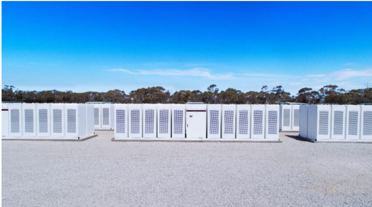
FIGURE 5 ILLUSTRATION OF CLOSE UP OF INDICATIVE BATTERY UNITS FOR ONE TYPE OF BESS (SOURCE: WWW.ENERGYAUSTRALIA.COM.AU/ABOUT-US/ENERGY-GENERATION/GANNAWARRA-BATTERY-STORAGE )
