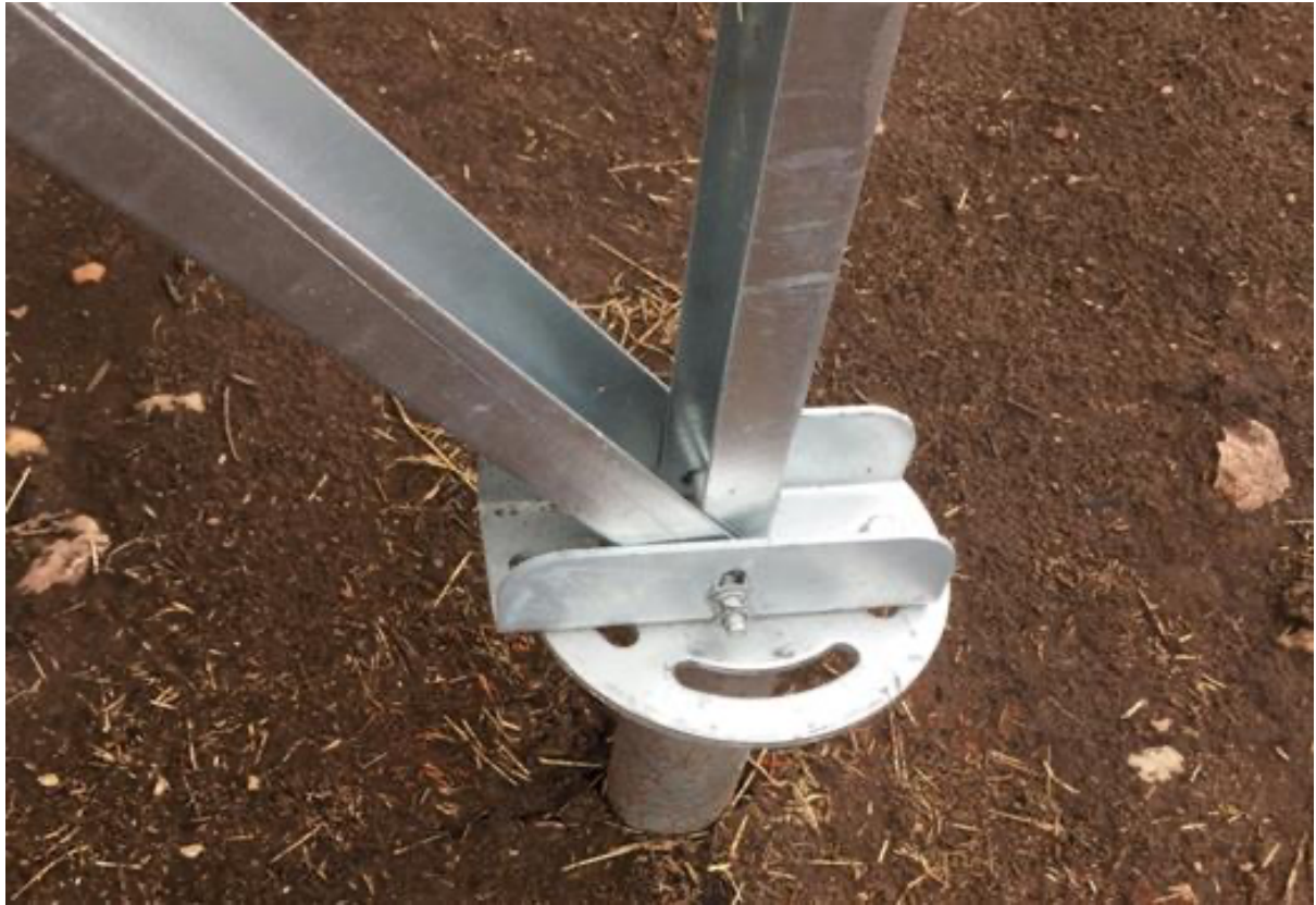
FIGURE 1 INDICATIVE SOLAR PANEL FOOTINGS
