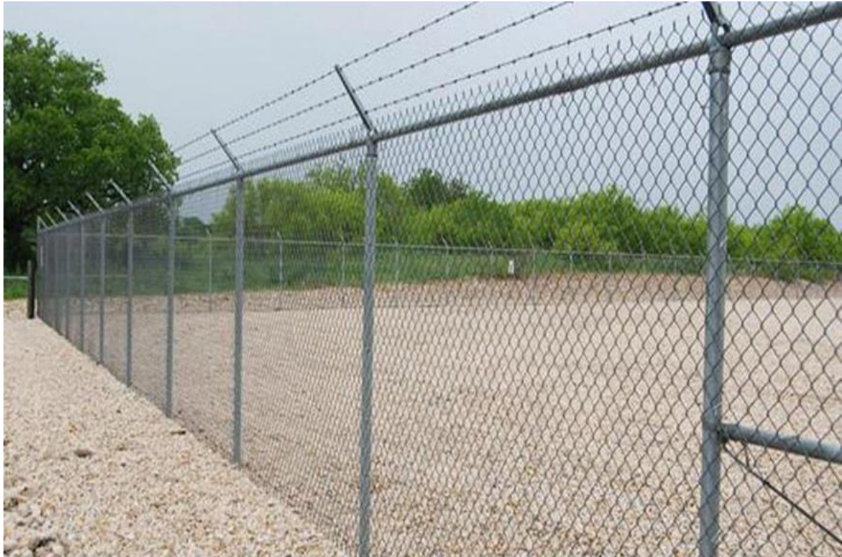
FIGURE 9 EXAMPLE PERIMETER FENCING
