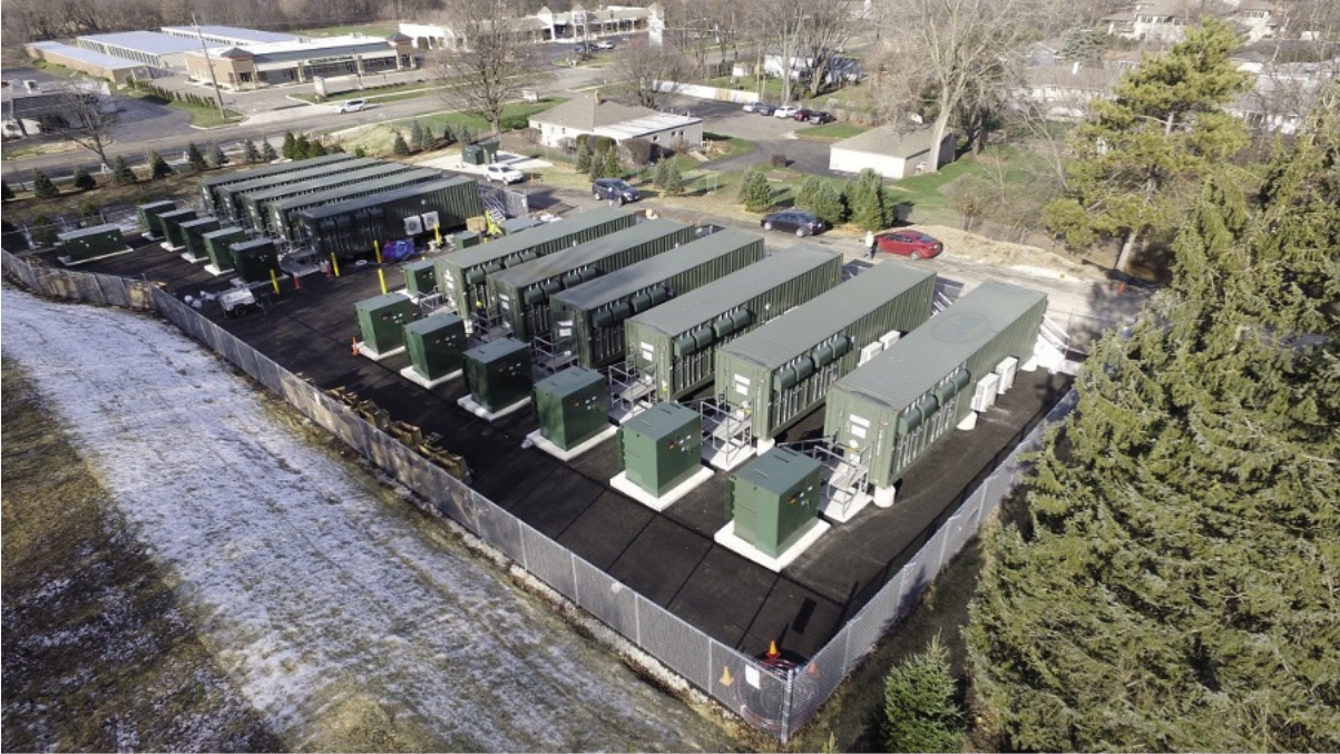
FIGURE 6 ILLUSTRATION OF CLOSE UP DETAIL OF INDICATIVE BATTERY UNITS FOR ANOTHER TYPE OF BESS (SOURCE: PV MAGAZINE)
