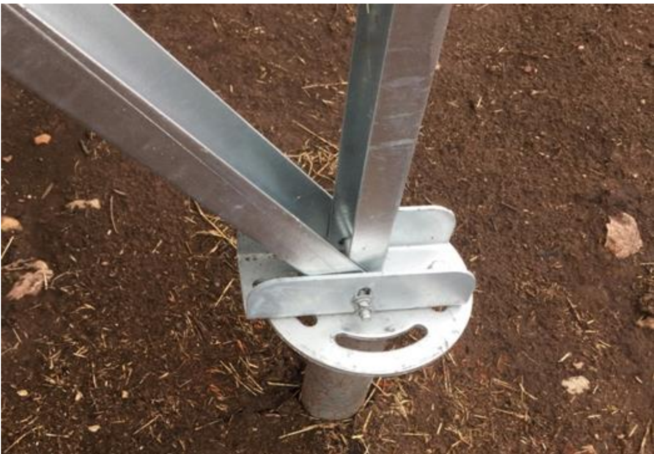
Figure 3-1: Example of Ground Mounting Arrangements
