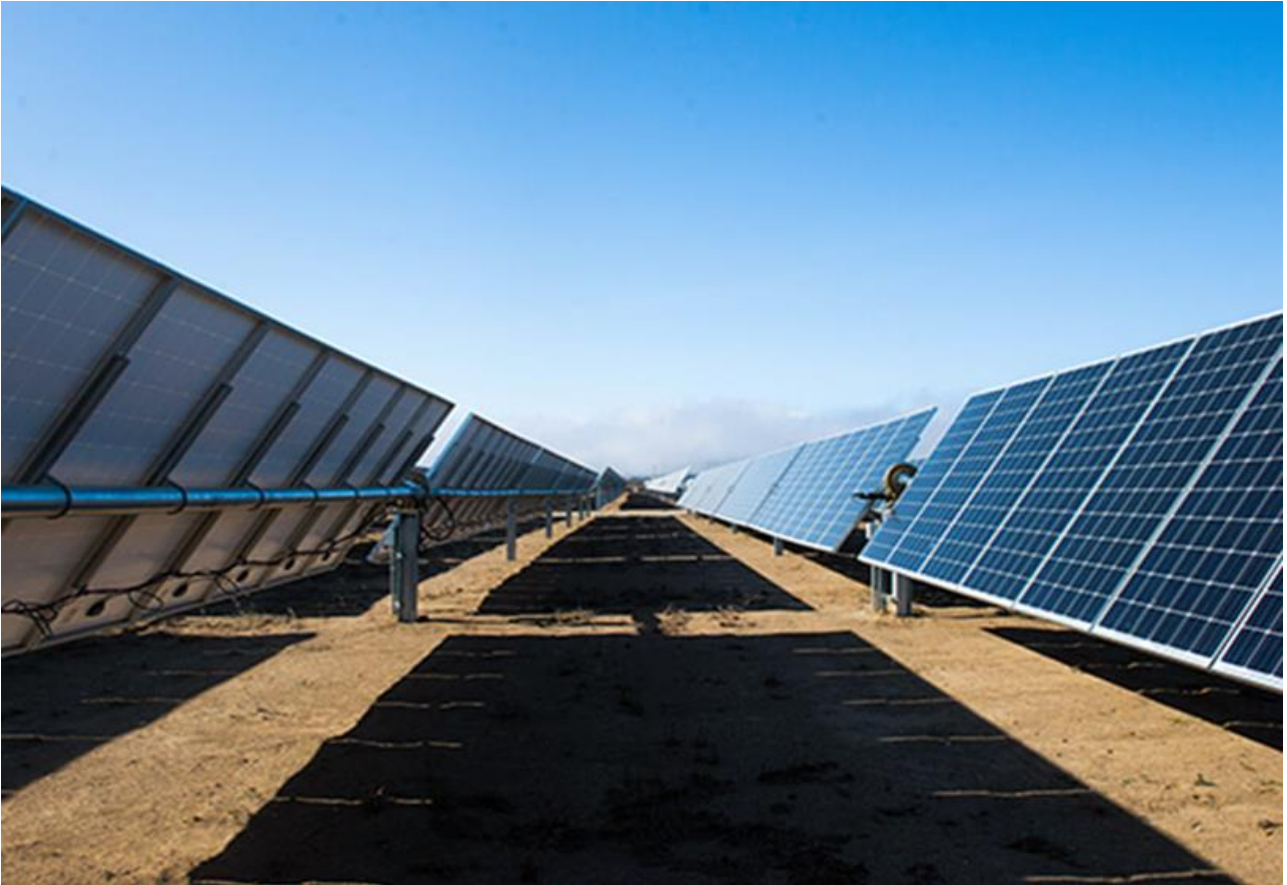
Figure 3-2: Example of Tracking Solar PV panels
