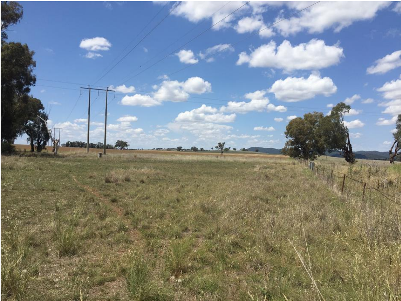
Figure 1-3: Existing Electrical Infrastructure in the Area
