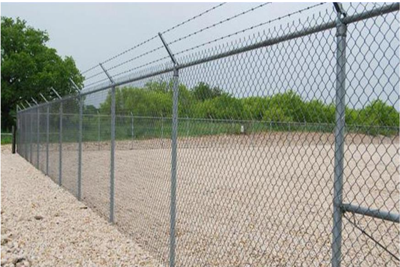
Figure 3-6: Example Security Fencing (Chain Link Security Fence)
