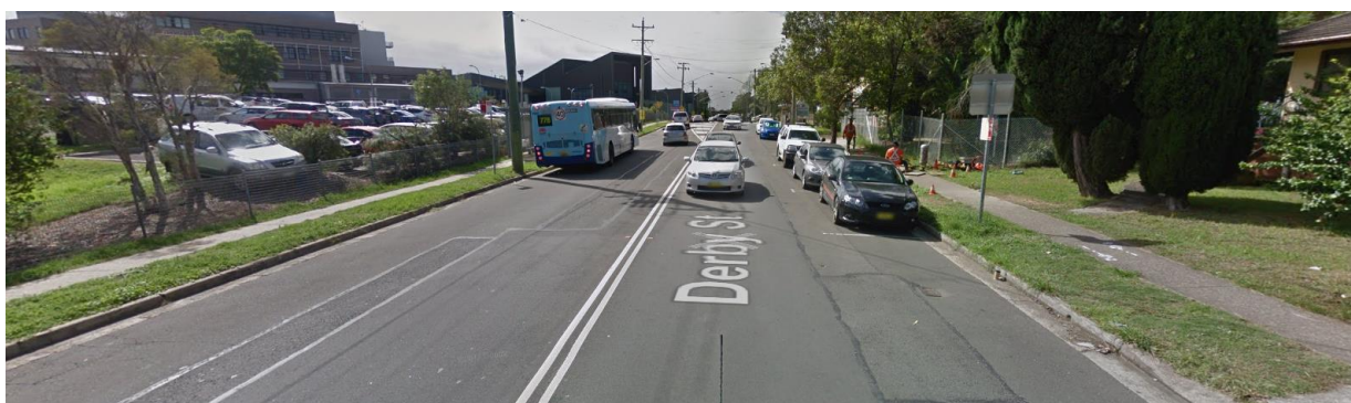
Figure 10 – Streetview of Dorby Street, Eastbound (Source: Google)
