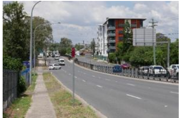
Figure 24. Parker Street. The new apartment building on the right, opposite the Nepean Hospital Campus, is typical of the likely future character of Parker Street.
