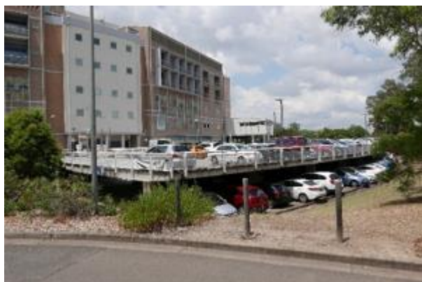
Figure 14: View south east, towards the existing car park within the western part of the Nepean Hospital Campus.
