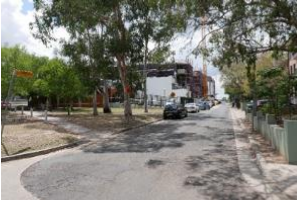
Figure 21. View north east, from the Wainwright Lane and Somerset Street intersection and rear of Kingswood shops.
