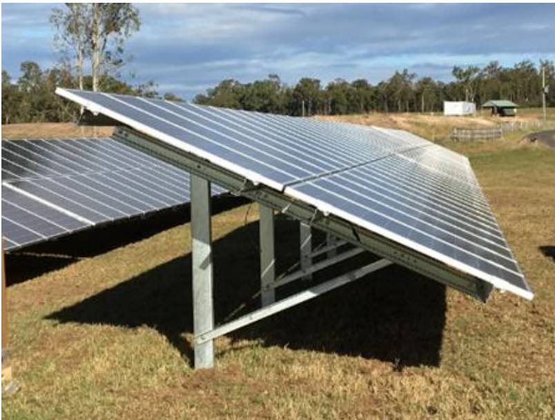
Figure 2-4: Example Ground Mounting Arrangements
