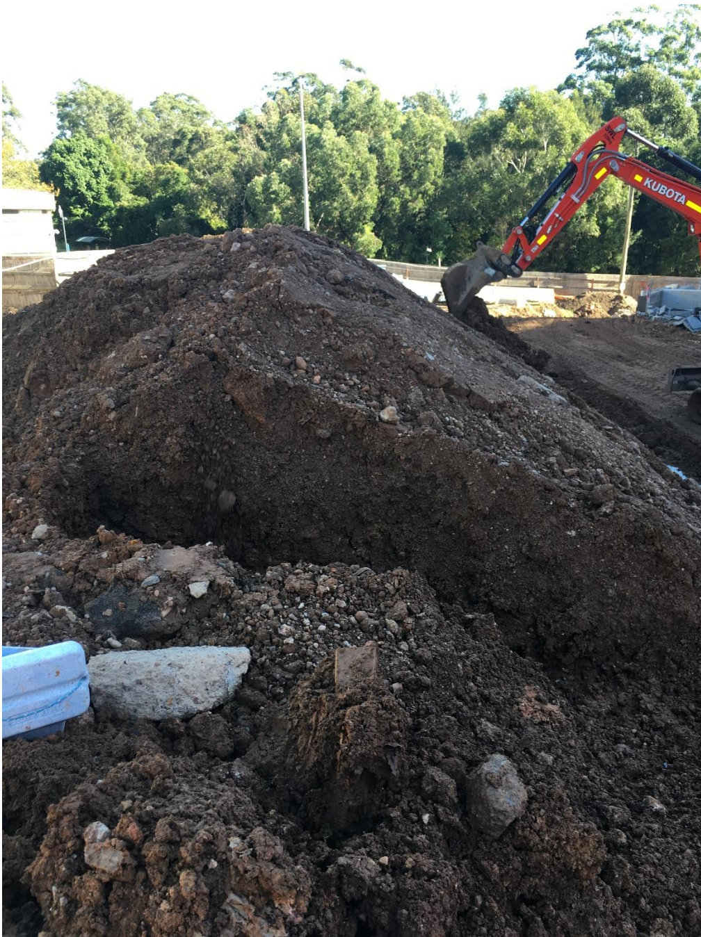
Stockpiled soil material (SP1) looking NW as observed 15.06.20
