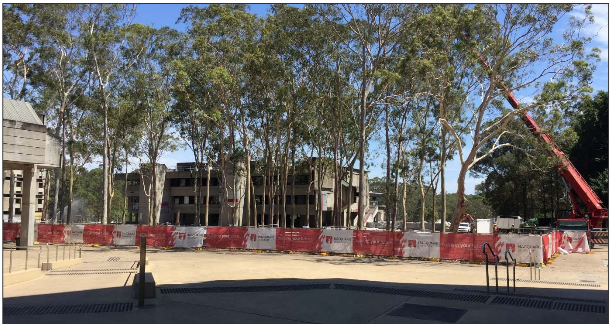
Figure 4 | View of the site from Wally's Walk – Central Courtyard in the foreground and recently demolished Campus Hub in the background (Source: Department)
