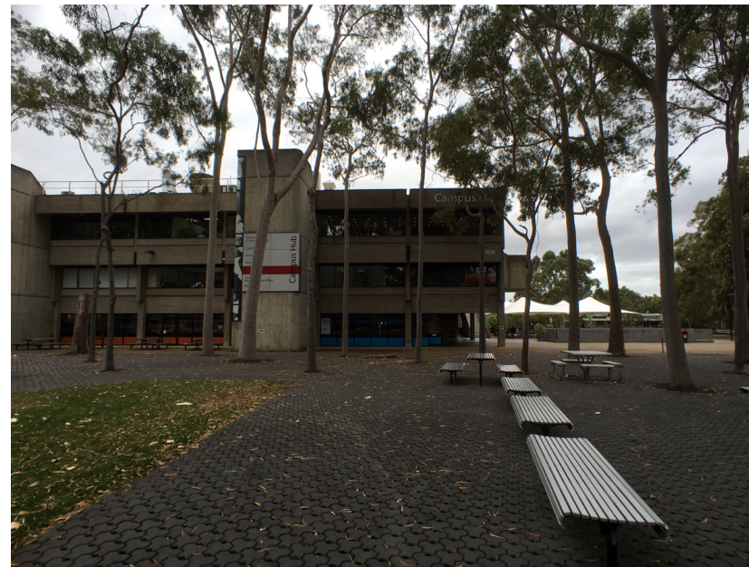
C10a – Stair towers interruptive to the Central Courtyard
