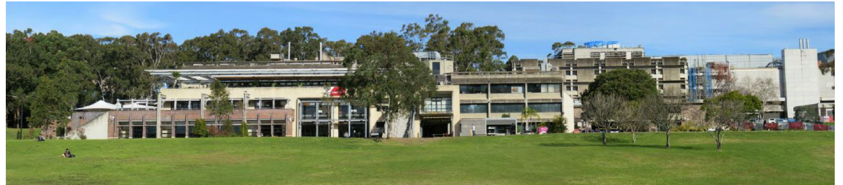
Building C9A, designed by Dick-Smith & Associates and built in c. 1970 was considered of 'Low' Legacy Value and was not a primary element of the Central Courtyard. Archival Recording of both C9a and C10a was conducted by Macquarie University prior to demolition.
