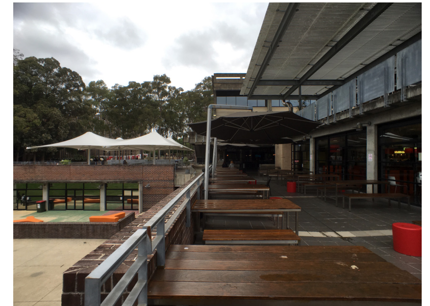
C10a – Terrace condition with multiple additions
