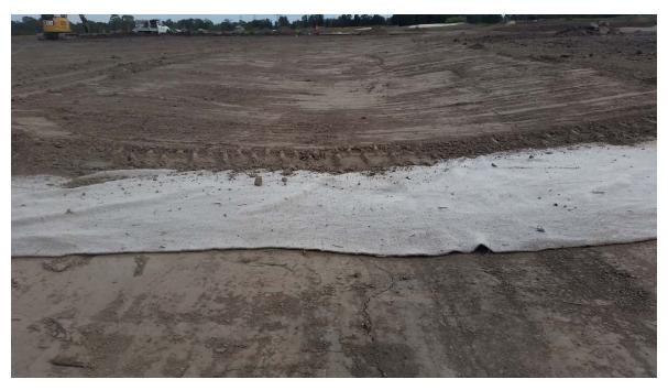
Figure 8 Membrane to be used in leachate dam and constructed wetland
