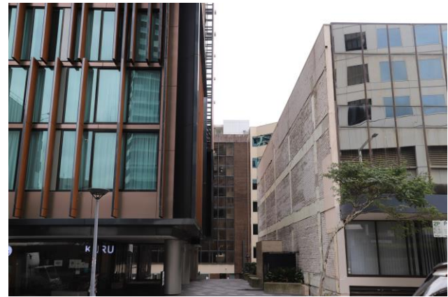
Picture 4 View north to Atchison Lane, along through site link
