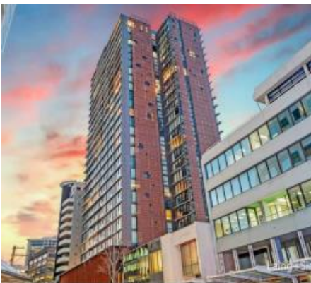
Picture 5 Eastern façade of 6-16 Atchison Street
