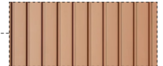
Metal Batten Cladding
