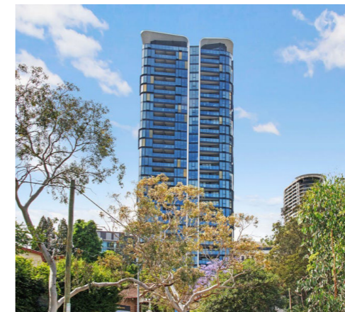
E) Embassy Tower
