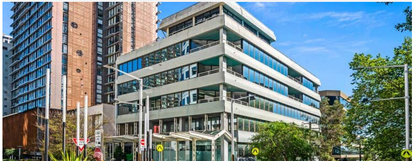
Figure 3 – Existing Development at 22 Atchison Street
