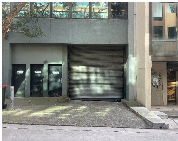
Figure 16 – Entrance to basement carpark to the rear of No. 22. Difference in level between No. 20 can be seen.
