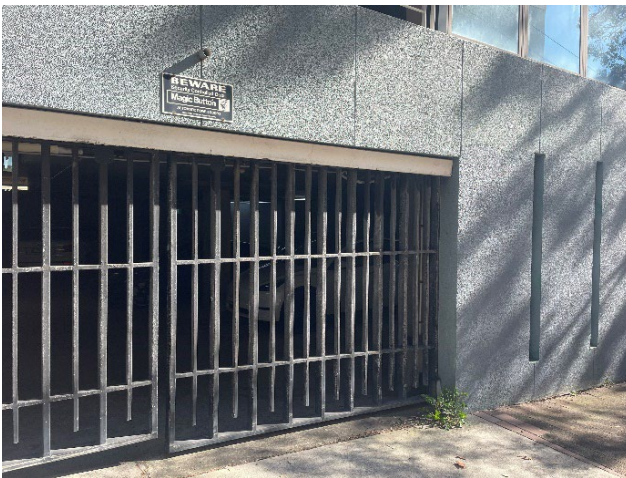
Figure 19 – Mitchell Street entrance to basement carpark of No. 22.
