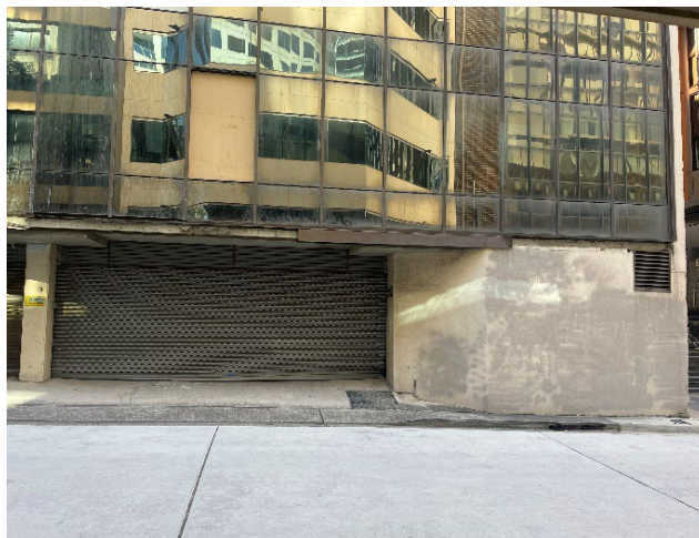
Figure 15 – Entrance to basement carpark to the rear of No. 20, showing drainage.
