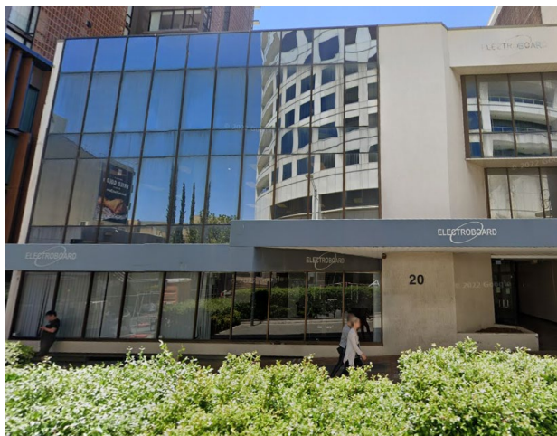
Figure 13 – Atchinson Street frontage, No. 20.
